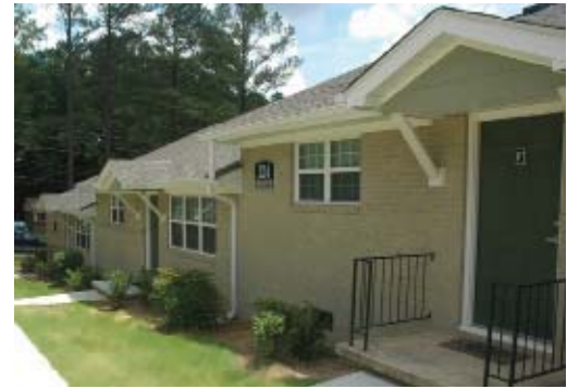
Newly rehabbed Glenbrook Crossing
