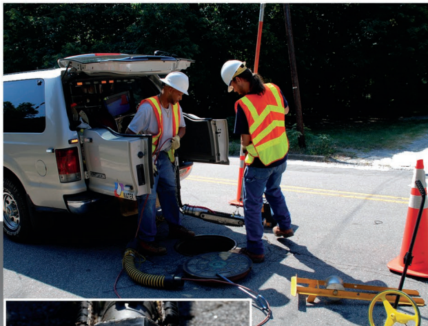
City of Raleigh CCTV crew preparing to inspect a sewer main for damaged or broken lines.
