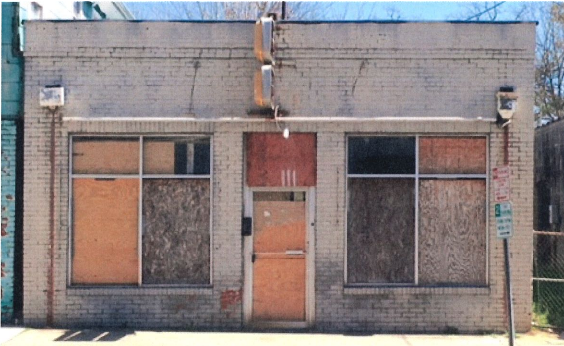
EXISTING FRONT FACADE - S. BLOUNT STREET
