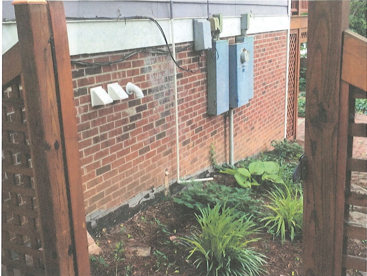
South wall of house, inside gate.
