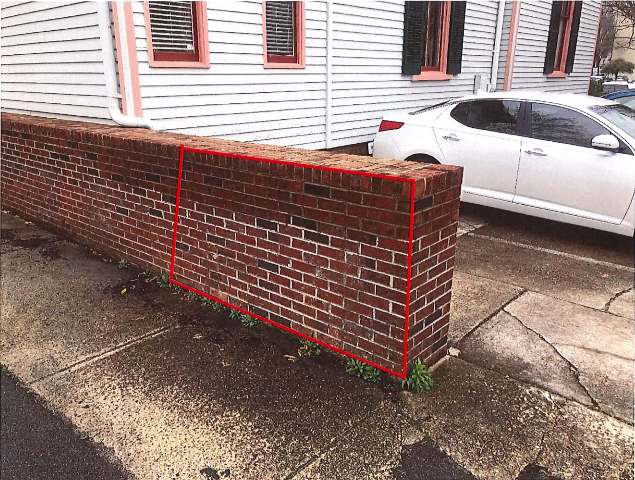
Minor Request #2 (Contd) - Backside of brick wall. Removal of area in red.
