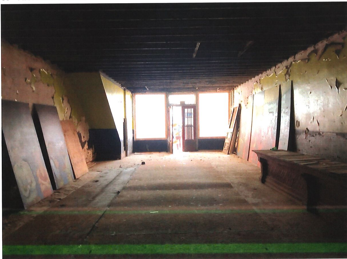
06 - First Floor Storefront Interior
