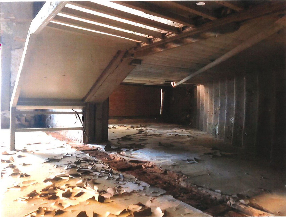
13 - Stairwell (photo turned 90 degrees counterclockwise)
