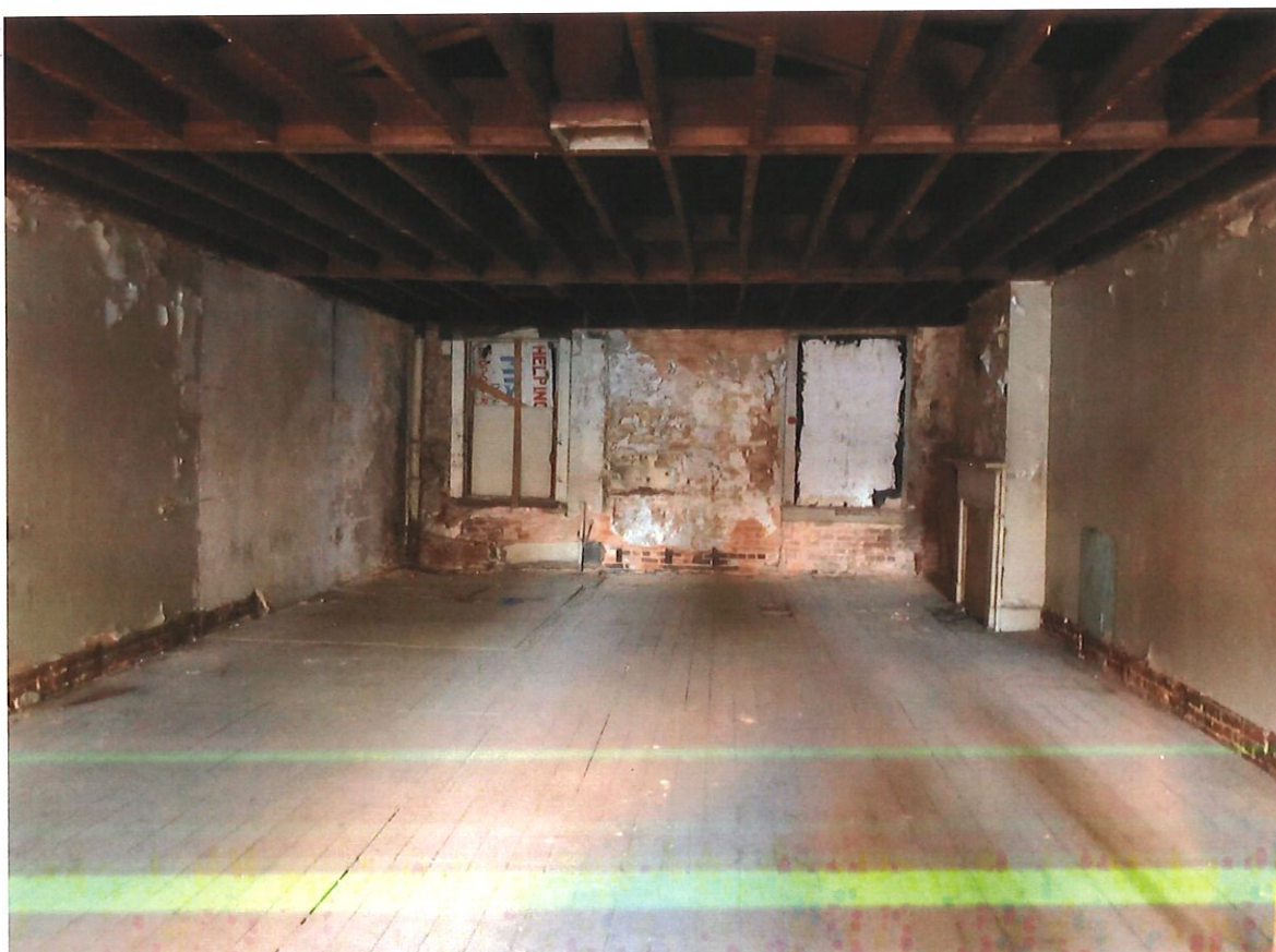
16 - Second Floor looking toward rear
