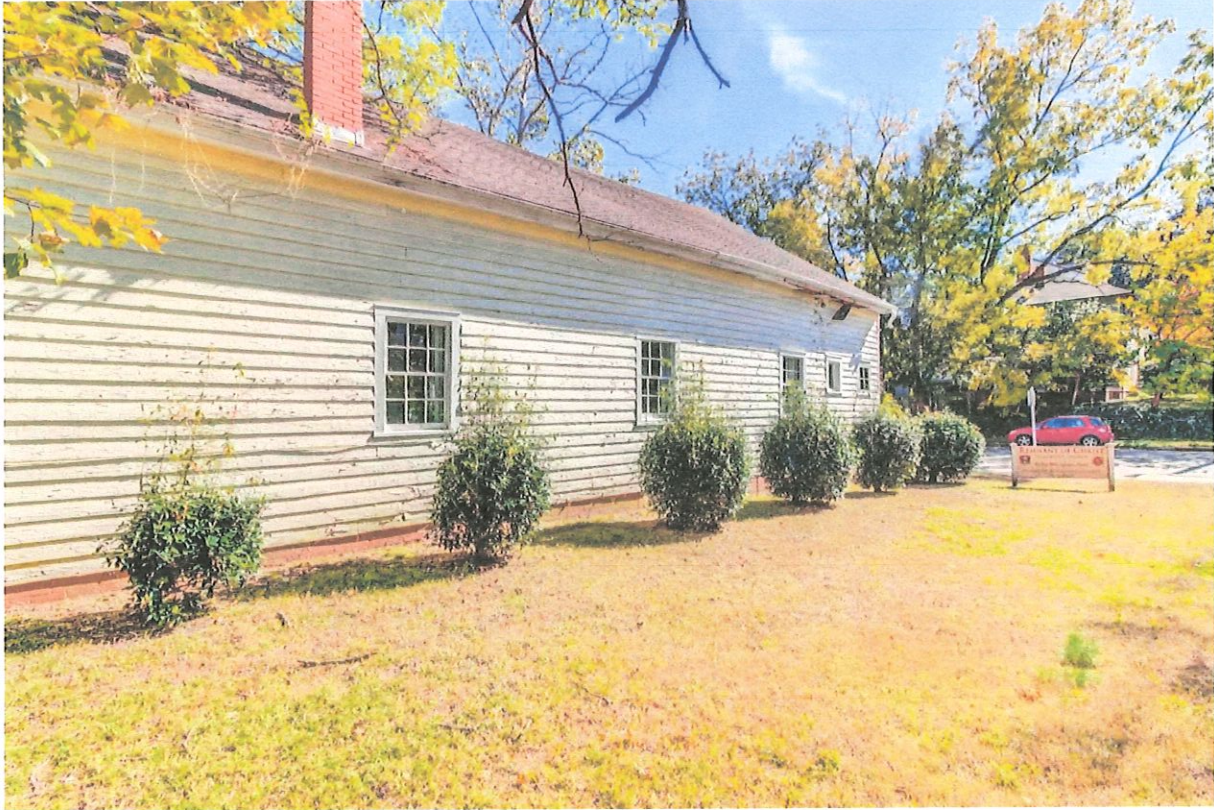
501 E Lane St view from northeast
