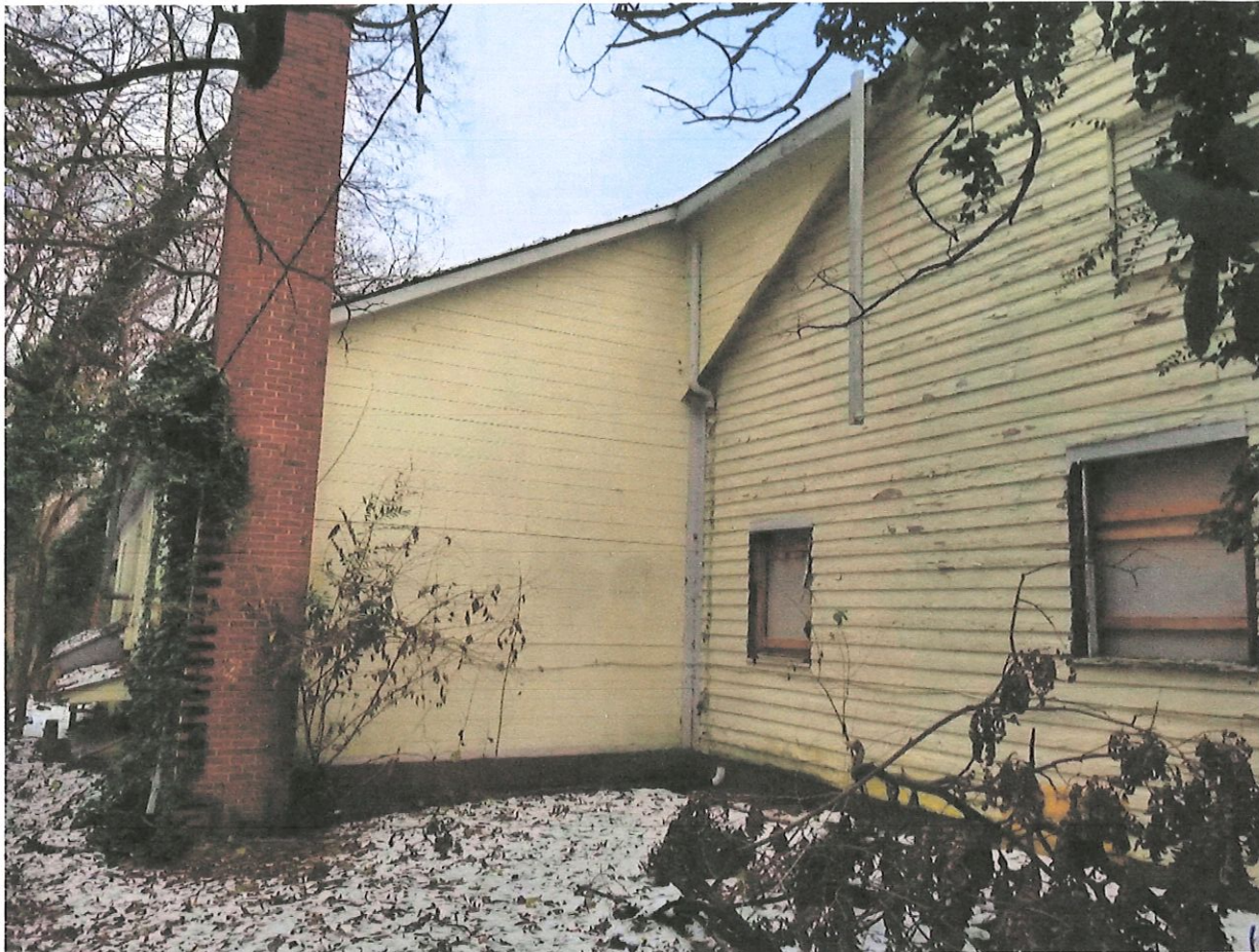
501 E Lane St view northwest corner of the lot, rear elevation
