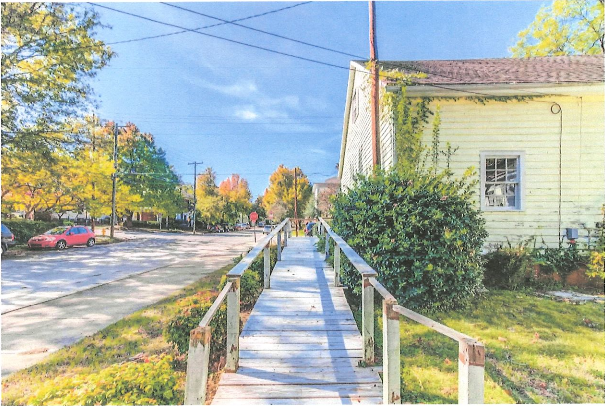
501 E Lane St view from east
