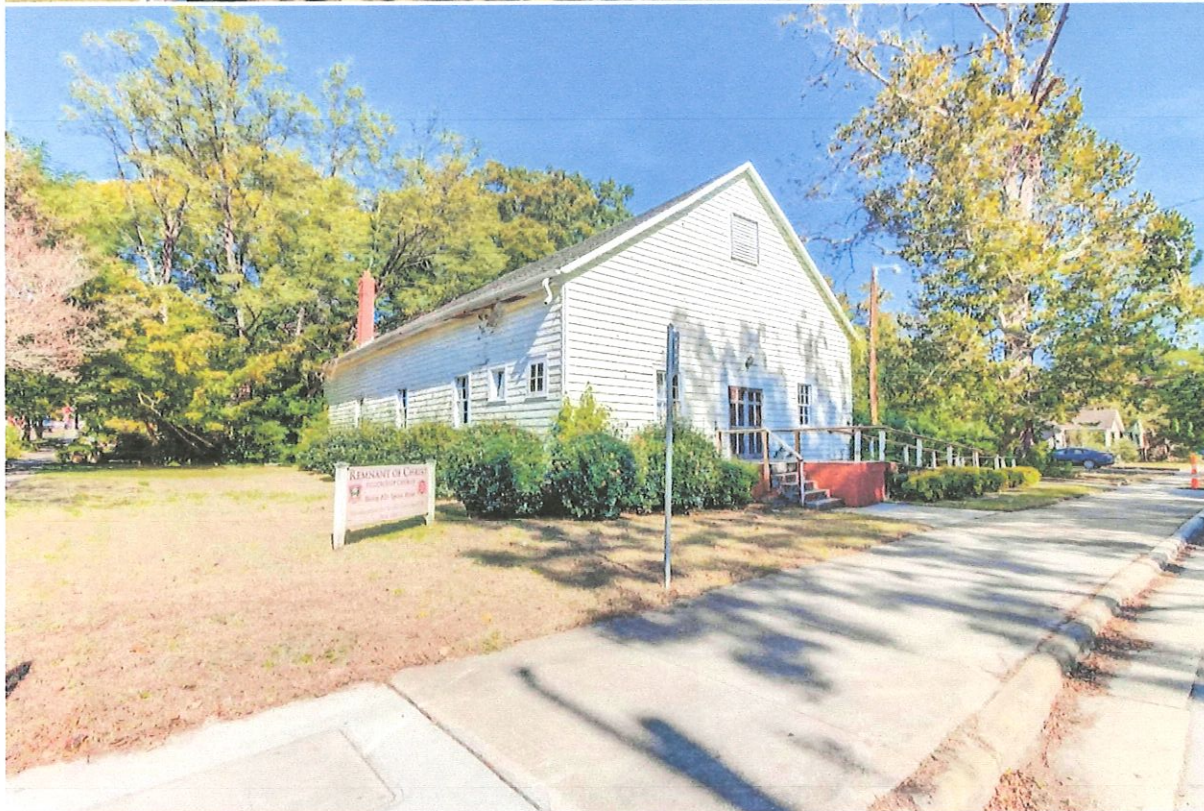
Different elevation views of 501 E Lane St view from southwest
