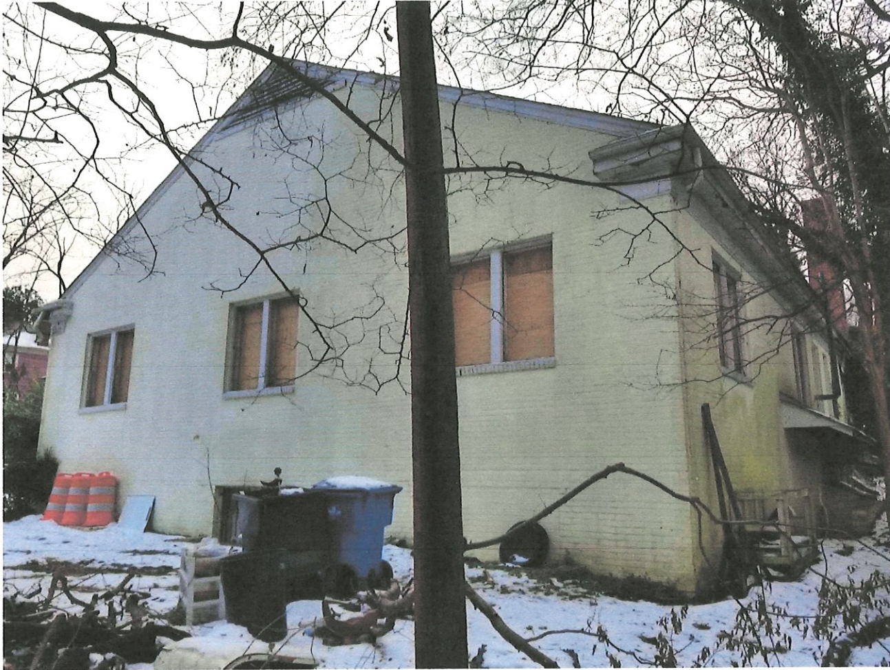
501 E Lane St view northeast corner of the lot, right elevation
