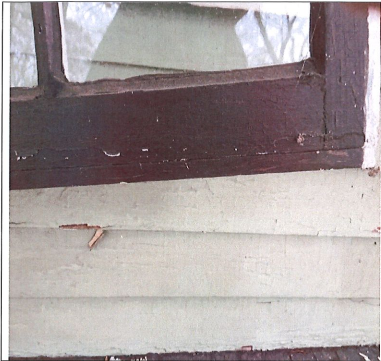
Bottom Rail With Added Wood Strip
