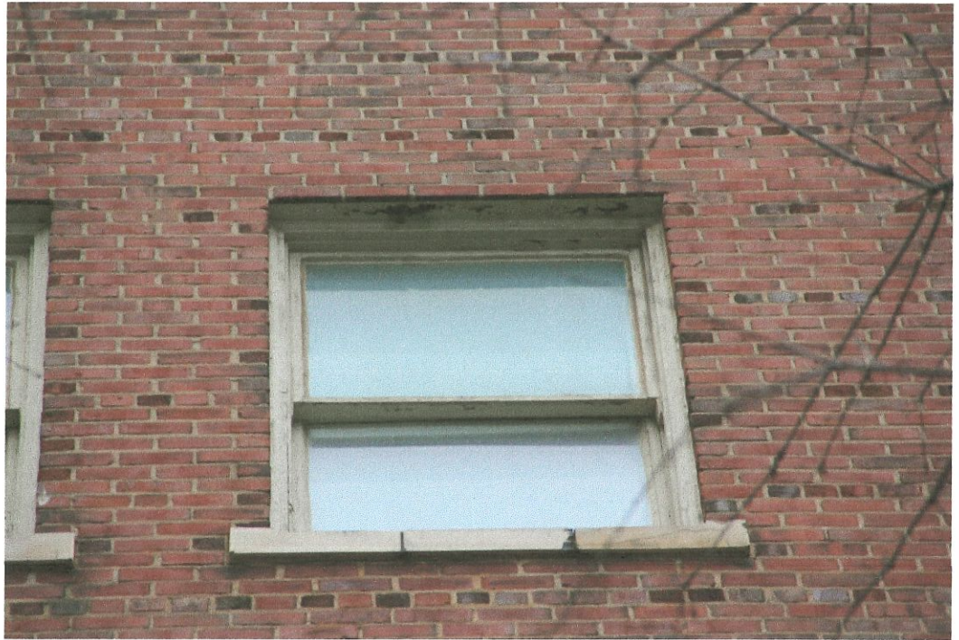
Typical window (floors 4 – 10)
