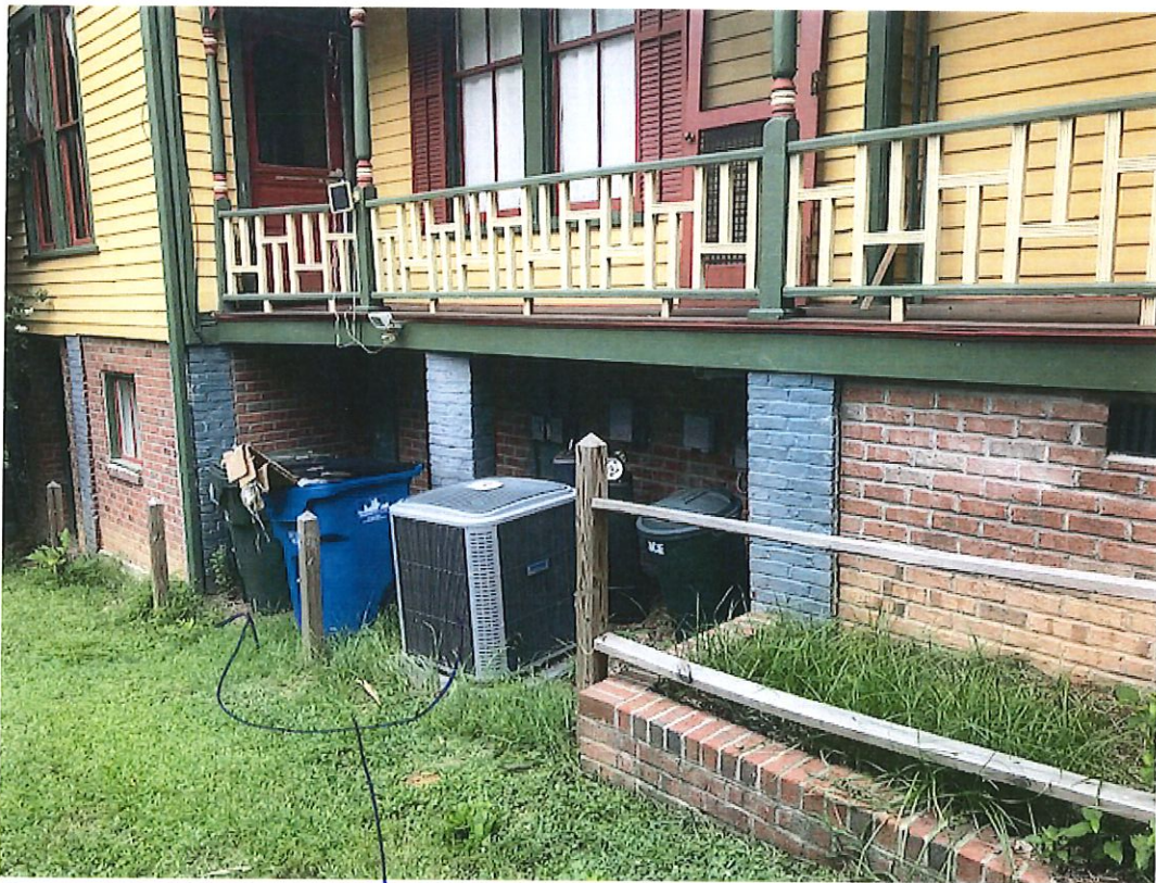
South Elevation Current A/C and future gas meter location
