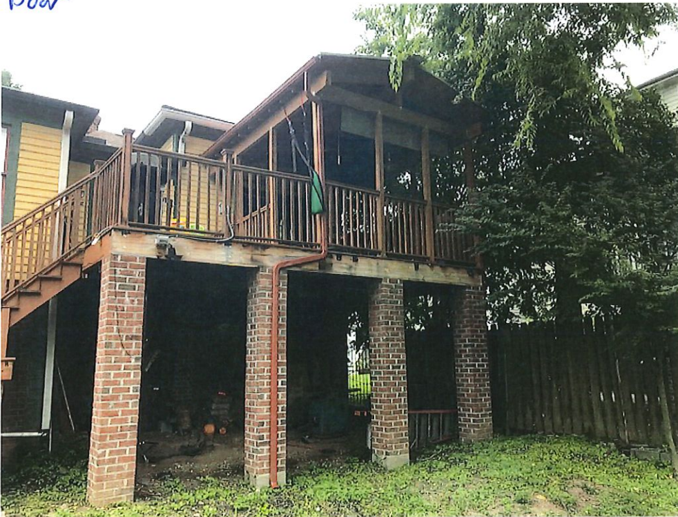
South West Back Corner
