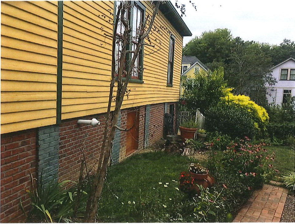
North Elevation facing backyard
