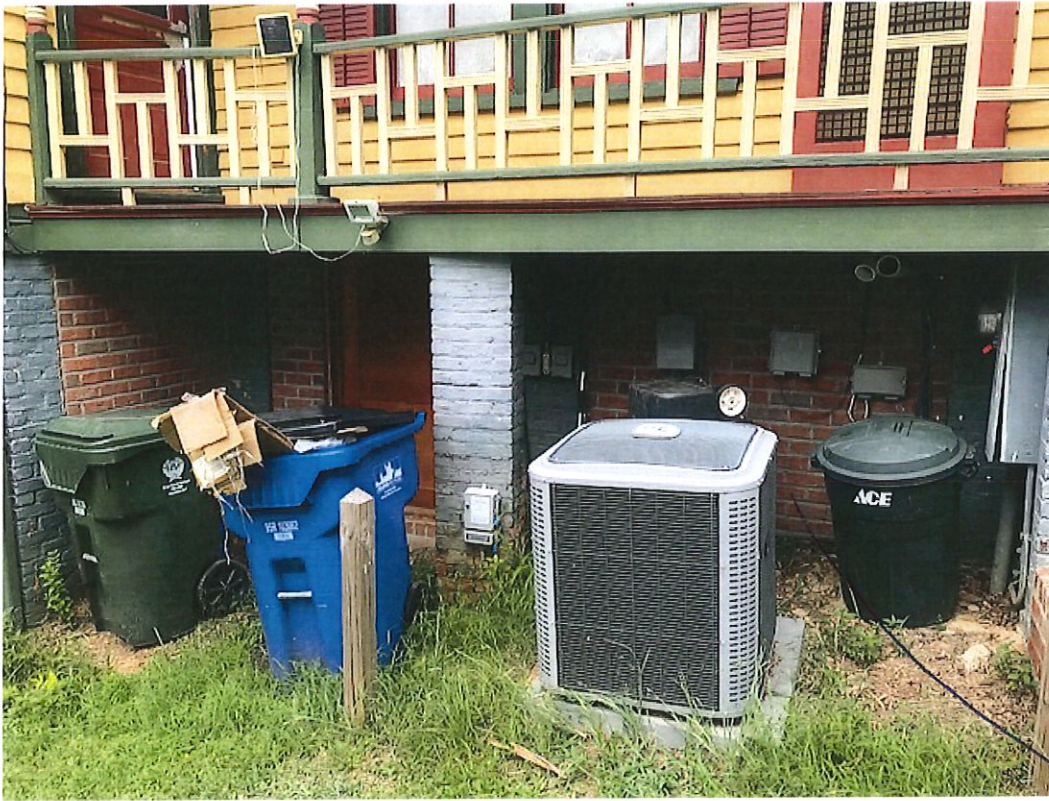
Close up of location of future gas meter and A/C unit
