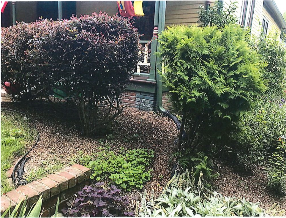
North East Corner /Brick retaining wall and porch edge
