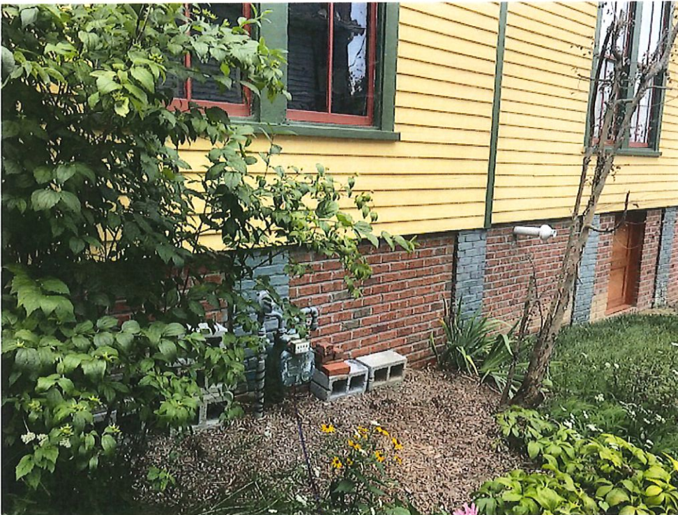
Gas Meter on North Elevation
