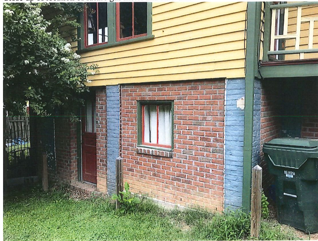
Current Door to Apartment Southern Elevation
