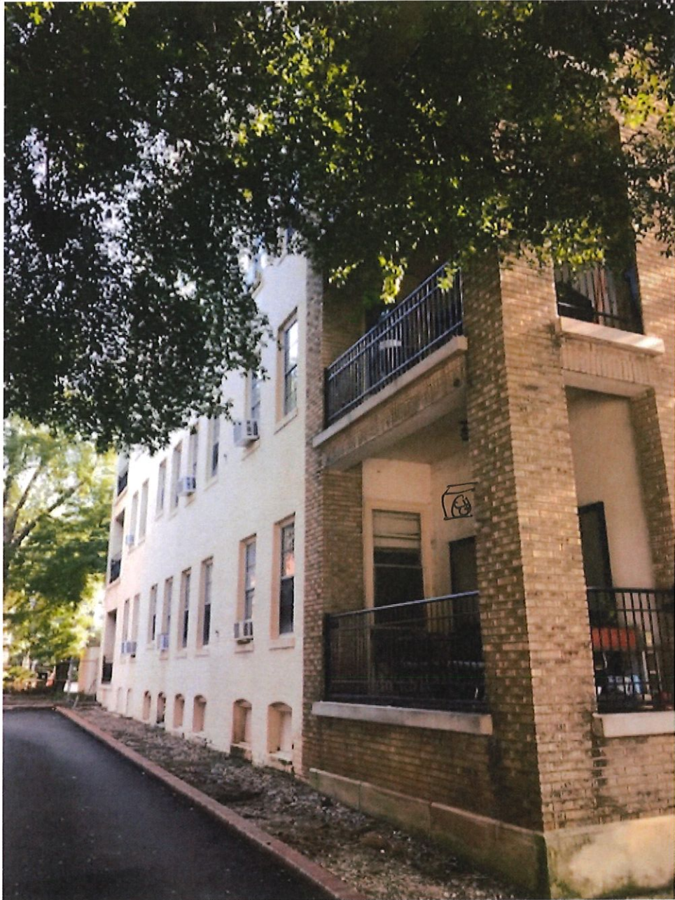
Left Side of Building.
