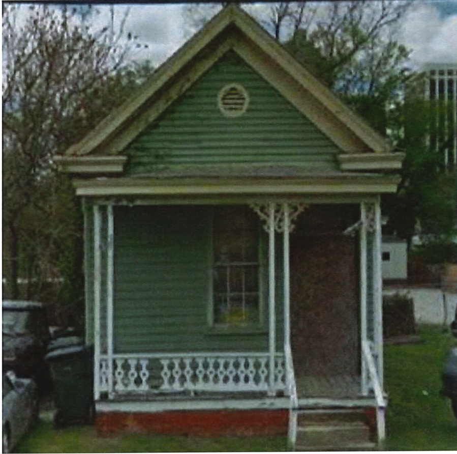
Front (east façade)
