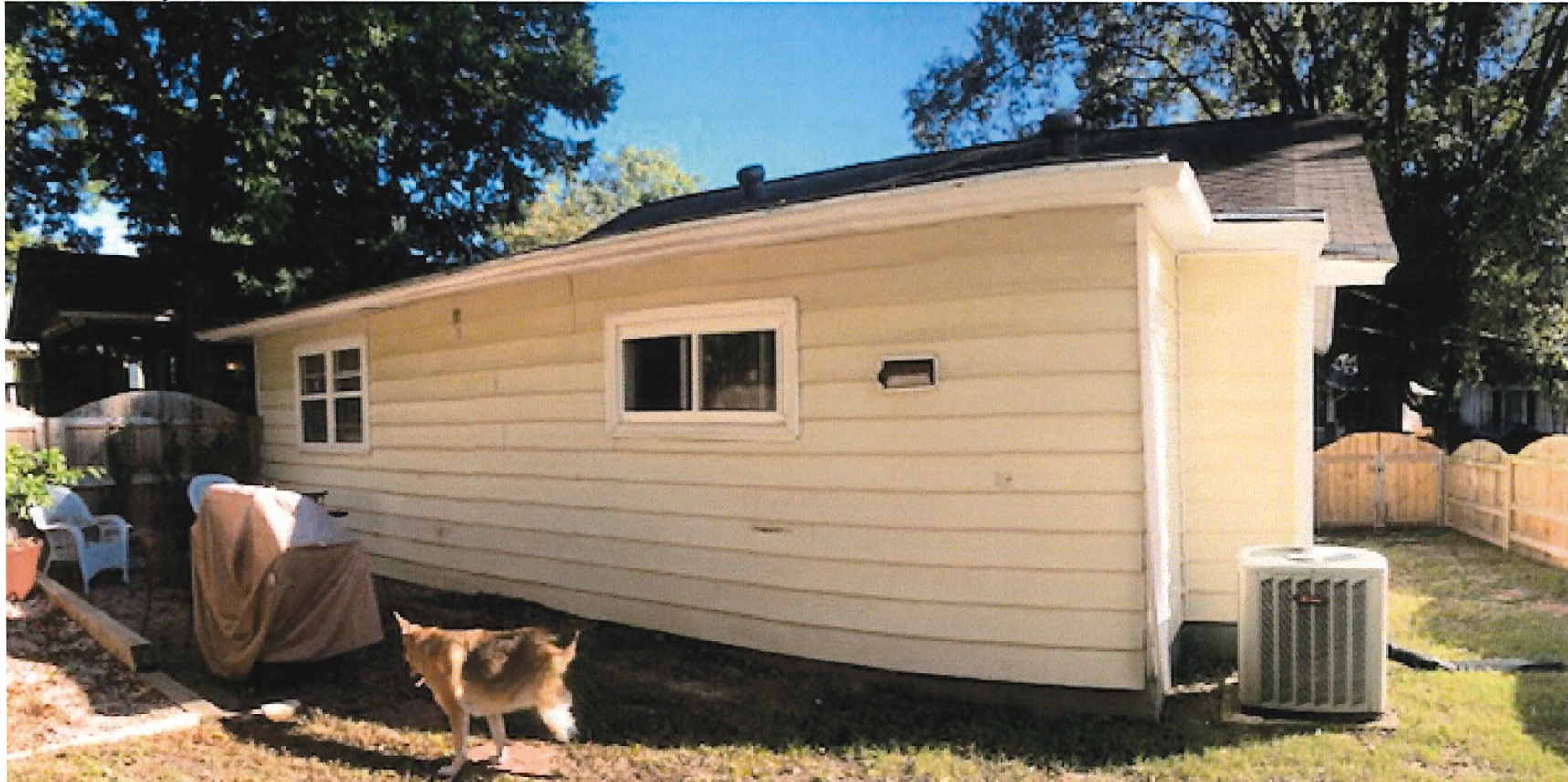
Current image of house rear:
