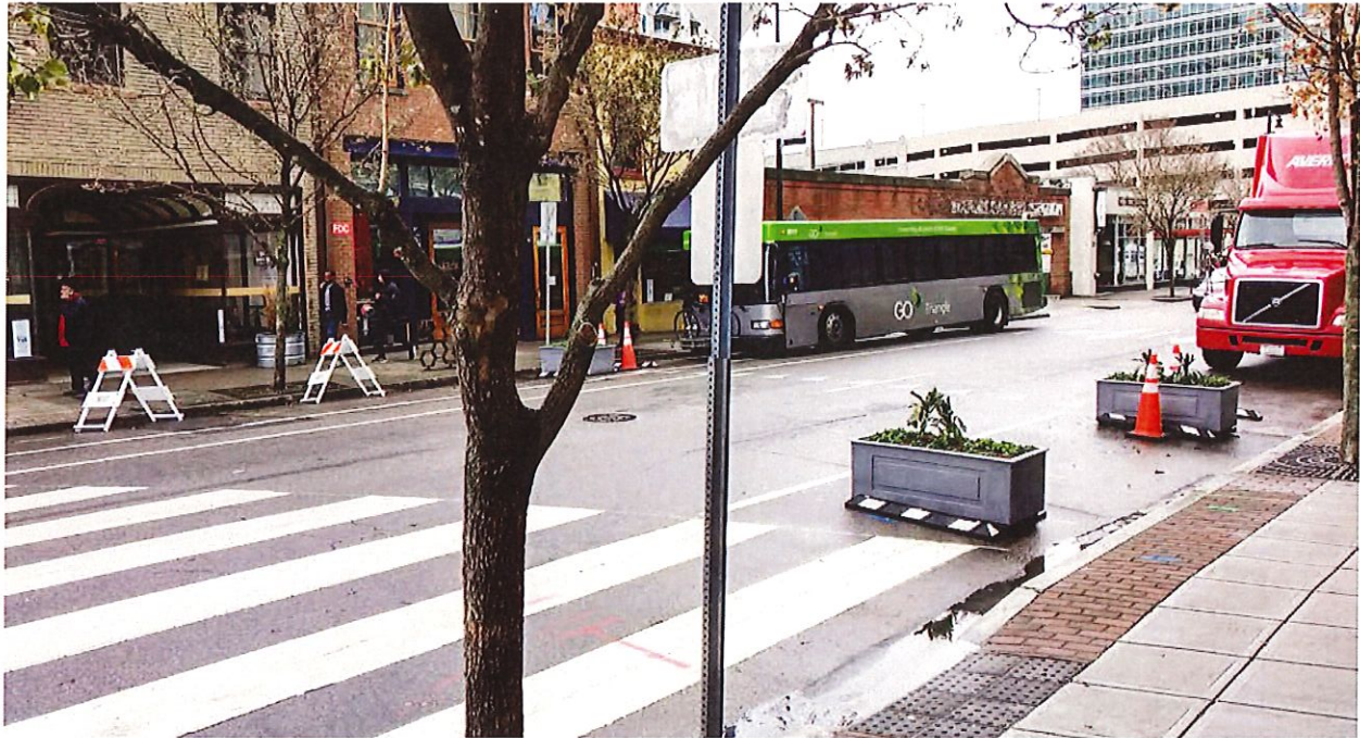
Image 3. The planters act as buffers on the south sides of the crosswalk and prevent buses and other vehicles from parking and blocking pedestrians' view of oncoming traffic. The murals and bike racks will be installed between the planters on both sides of Wilmington Street.
