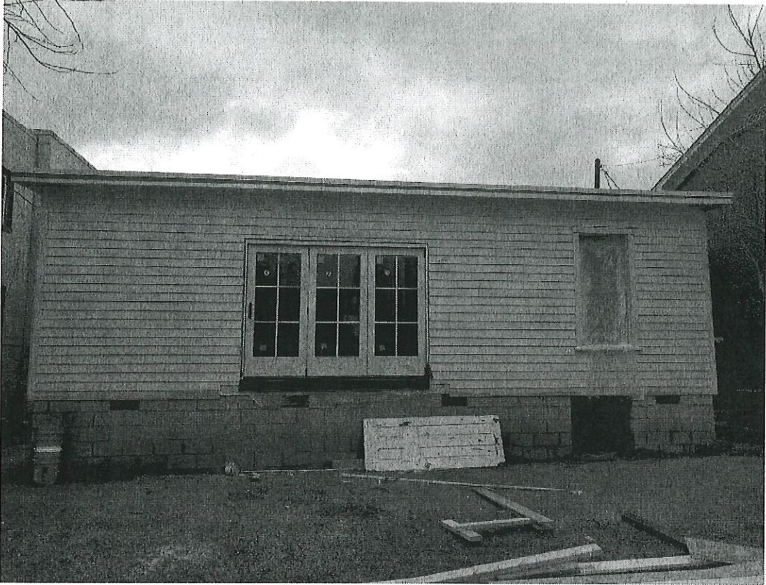
Steps have been removed, foundation has been repaired, and folding door has been added as part of the duplex to single family conversion. New siding was used to prevent a patchy look. Original COA application for 6x6 deck was based on contractors miscalculation of how much deck would be needed to support opening of folding doors which measure 10 feet wide.
