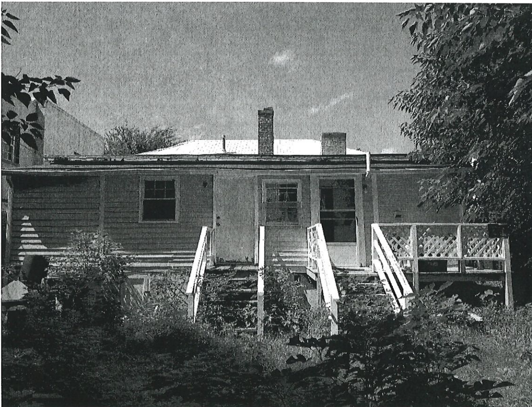
Previous rear elevation.
