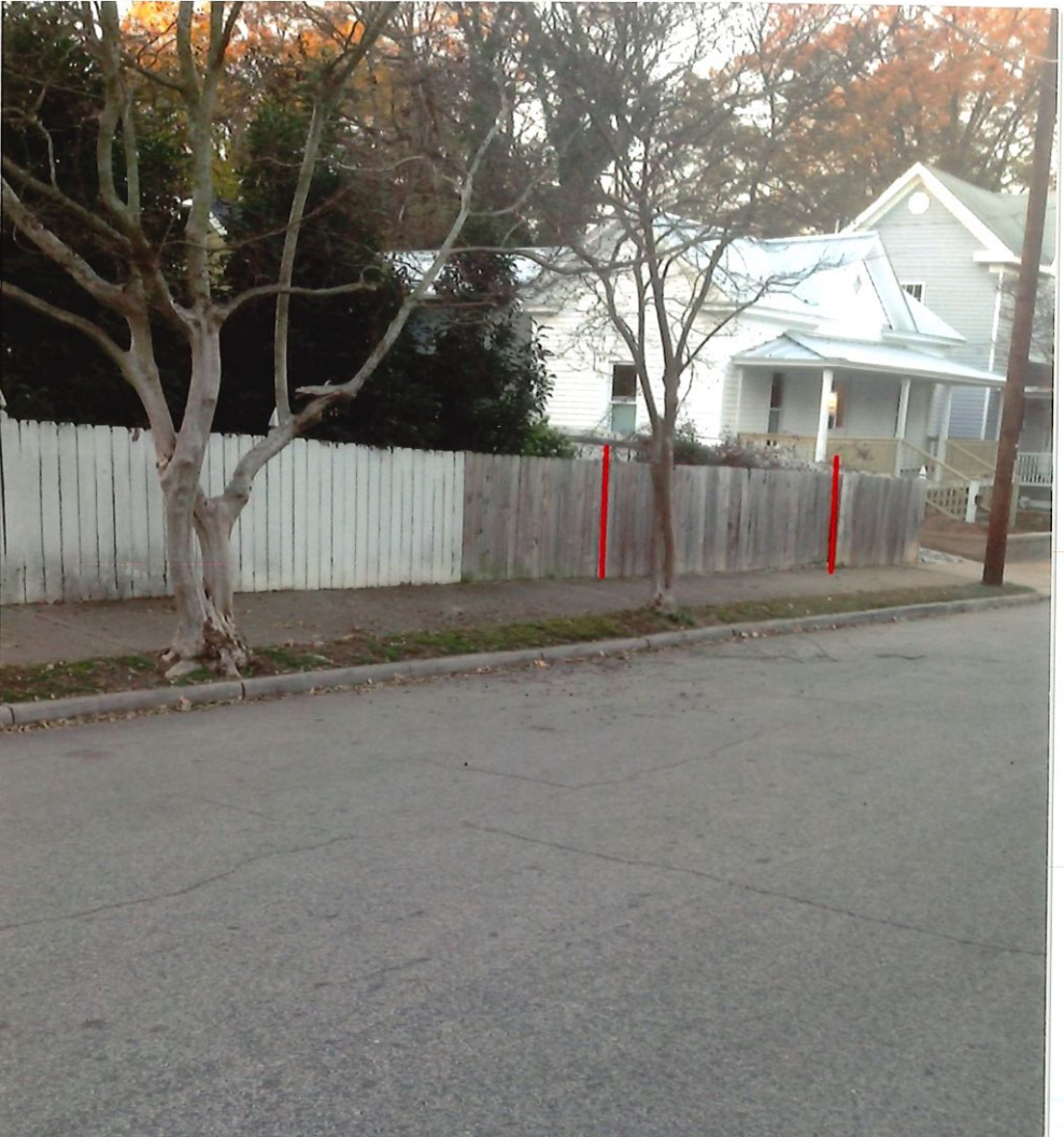
1100 DENVER ST, CURB CUT & FENCE REMOVAL (BETWEEN RED LINES)
