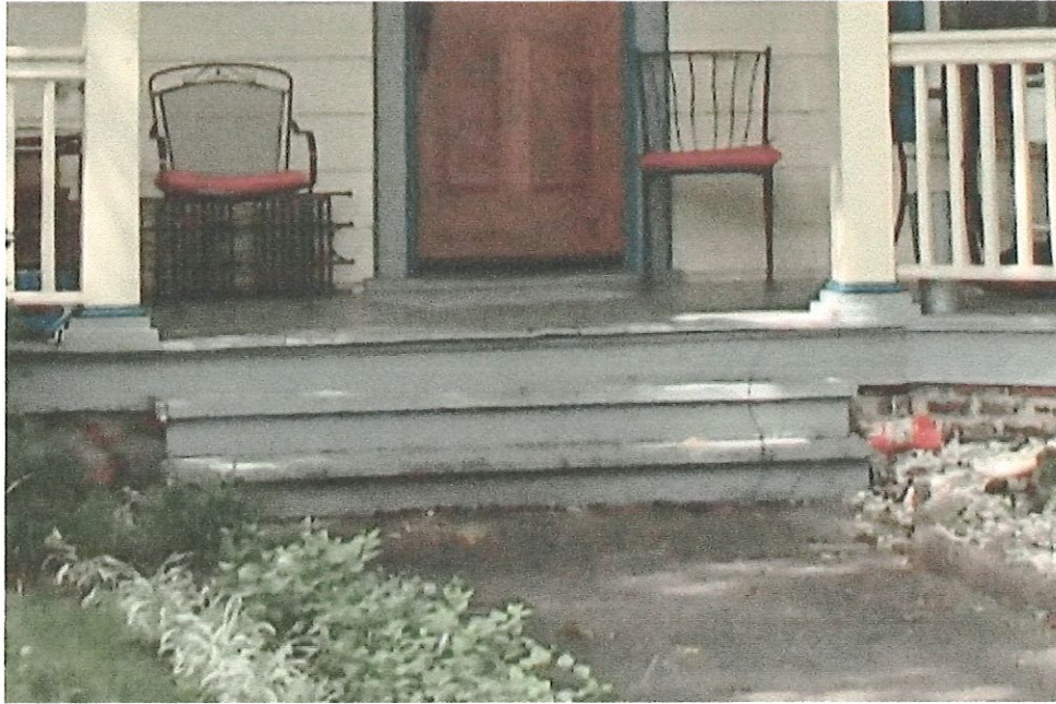
Existing wooden steps
