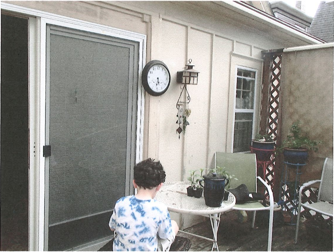
Board and batten siding on enclosed porch
