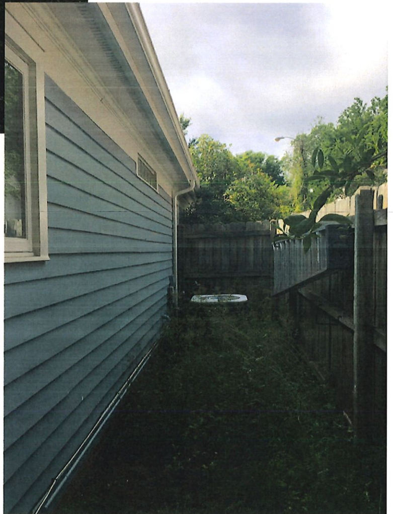
Existing side elevation and side yard
