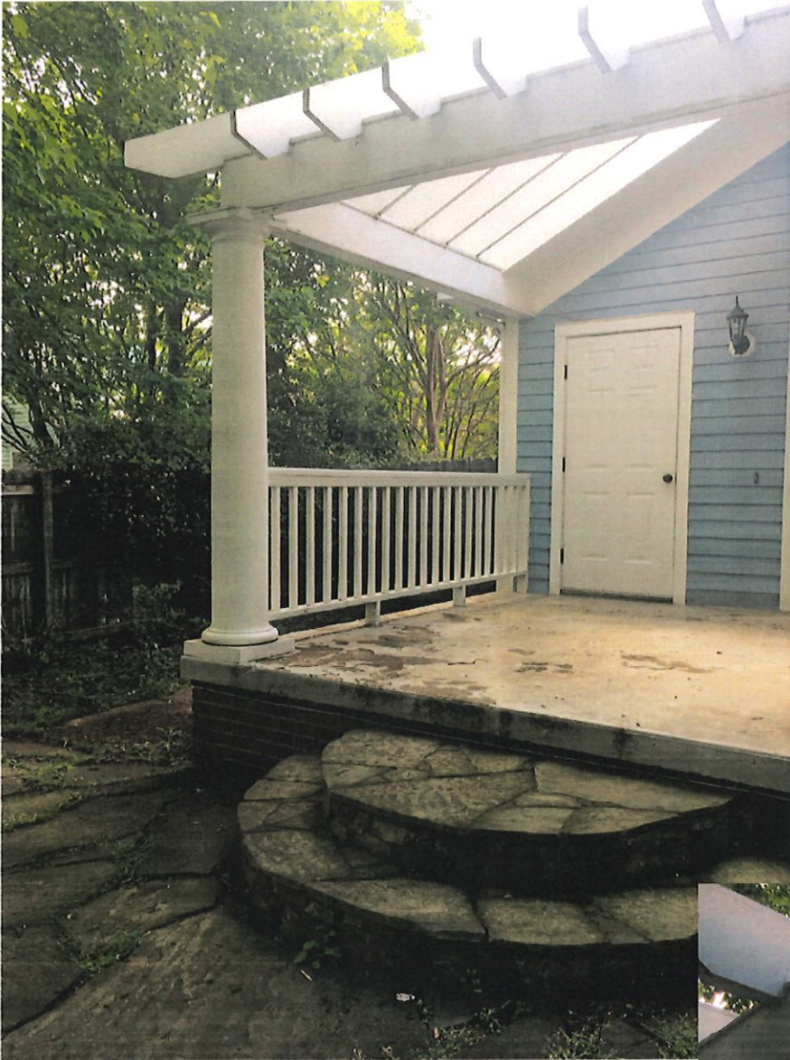
Existing Rear Porch and roof framing
