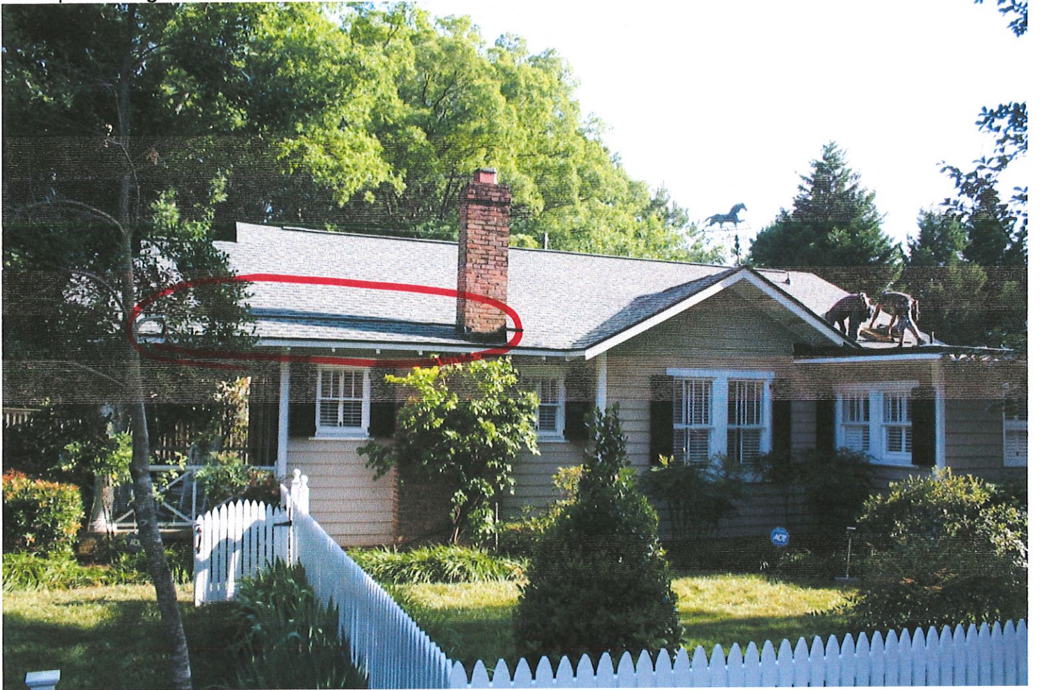
Example of Edge Intake Vent #5
