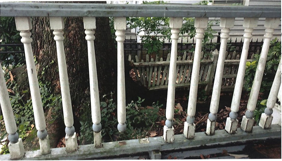
SPINDLE REPAIR AS NEEDED
