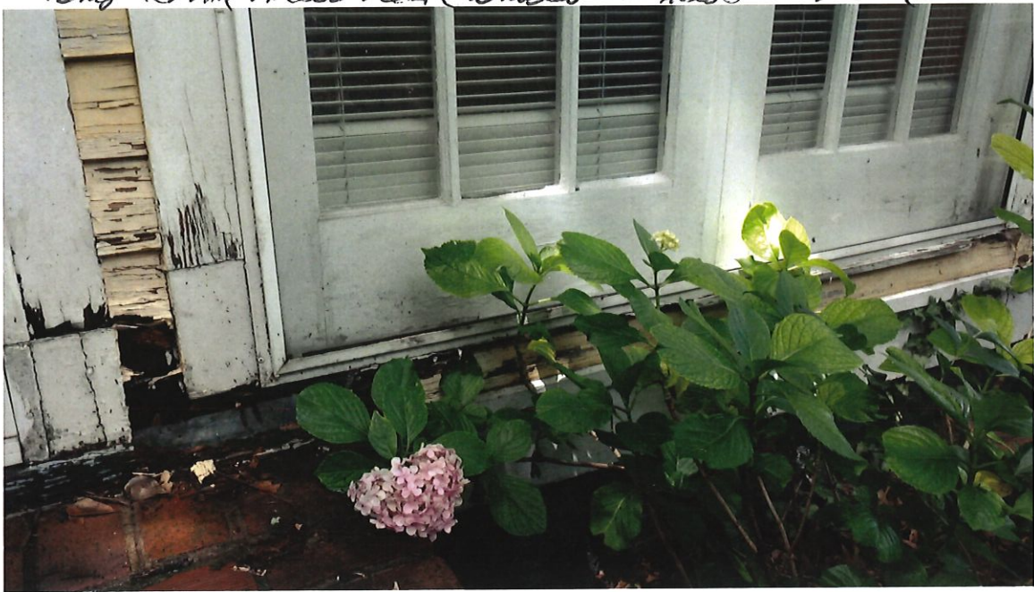
Siding REPAIR AROUND REAR WINDOW OF HOUSE 1st FLOOR
