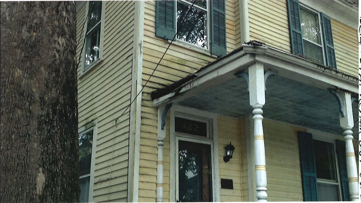
FASCIA & SOFFIT REPAIR ON FRONT LEFT CORNER OF PORCH.
