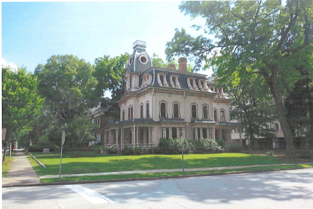
Existing Heck-Andrews House North & East Elevations From Corner Of North And Blount Streets
