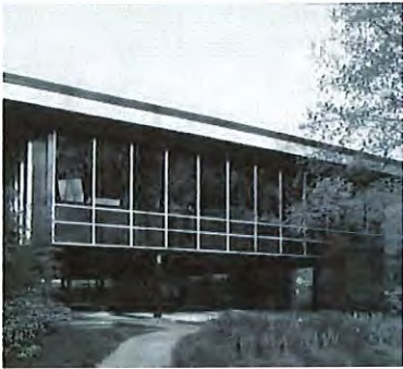
The curtain wall facade of this Raleigh landmark is characteristic of many mid-century modern office buildings which embraced large spans of non-loadbearing glass walls.
