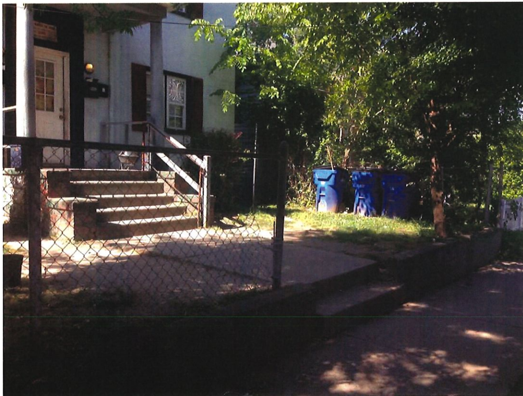
Front Porch & Sidewalk
