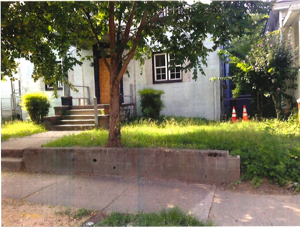
Front Porch & Sidewalk
