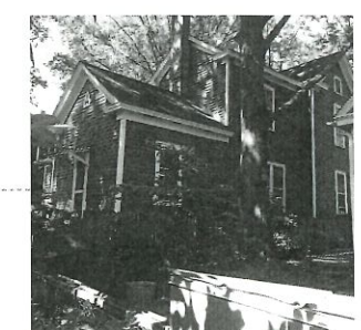
Photographs of Existing
