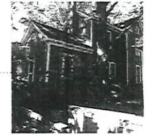
Photographs of Existing
