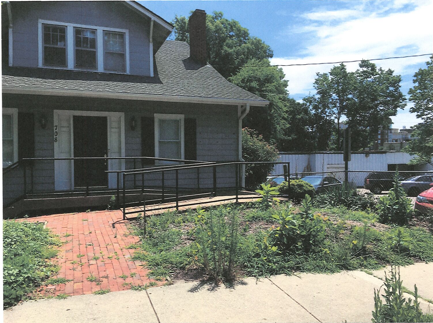
708 St. Marys Street, Raleigh NC 27605 existing conditions
