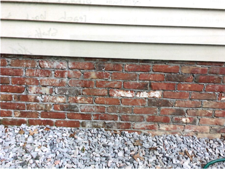
Brick at 515 N Boundary
