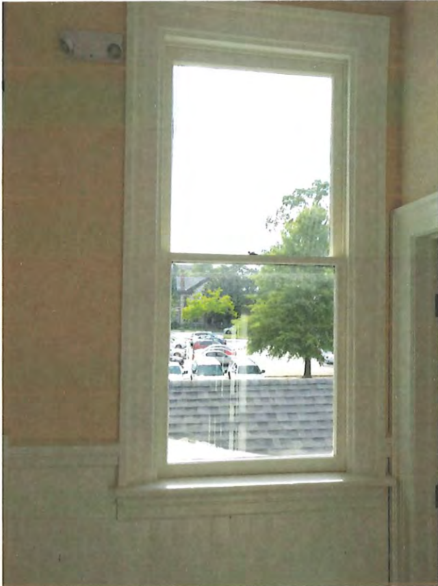
existing window . interior
