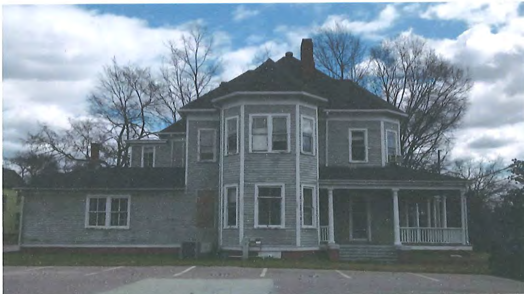
Photo of Exterior . West Elevation
