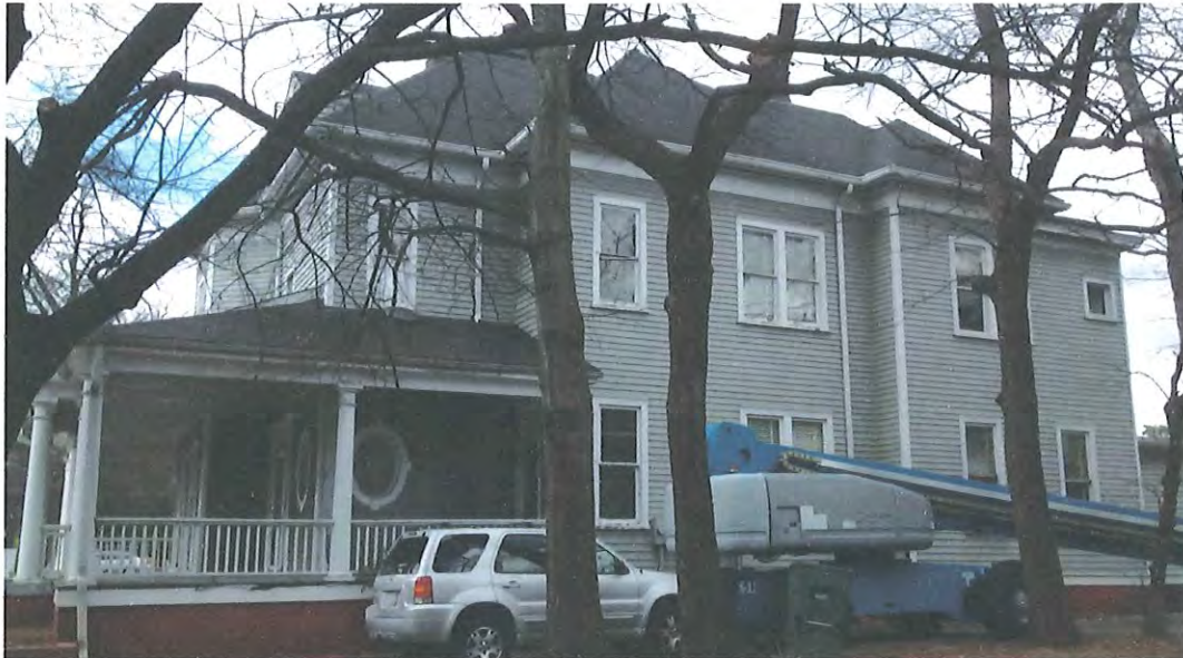
Photo of Exterior . West Elevation
