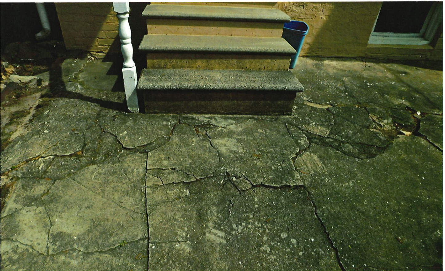
6 EXISTING CONCRETE PATIO @ STEPS
