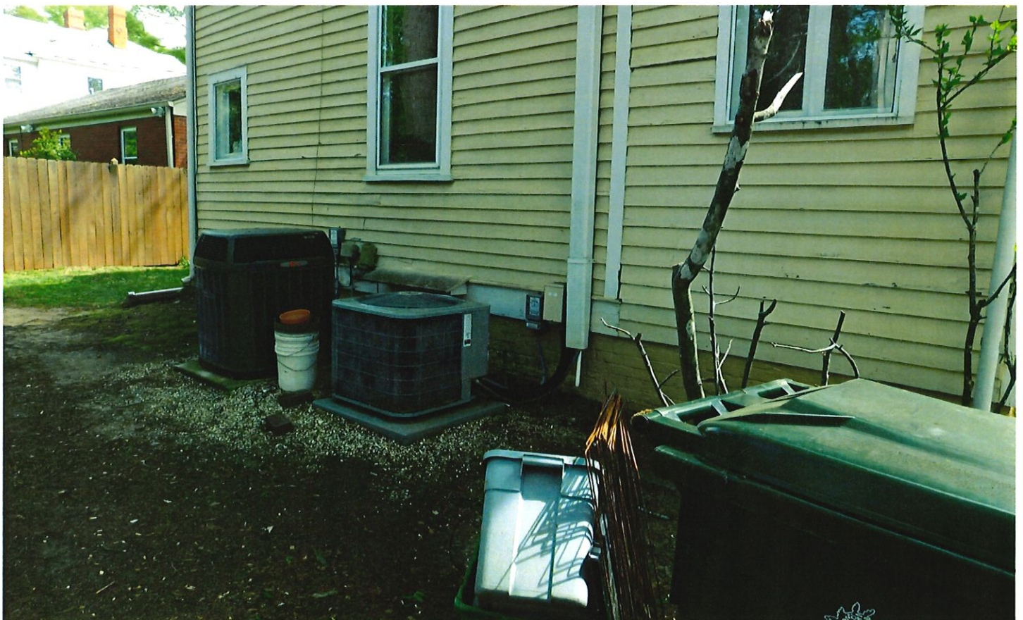
4 REAR OF HOUSE W/ HVAC EQUIPMENT & CANS TO BE SCREENED
