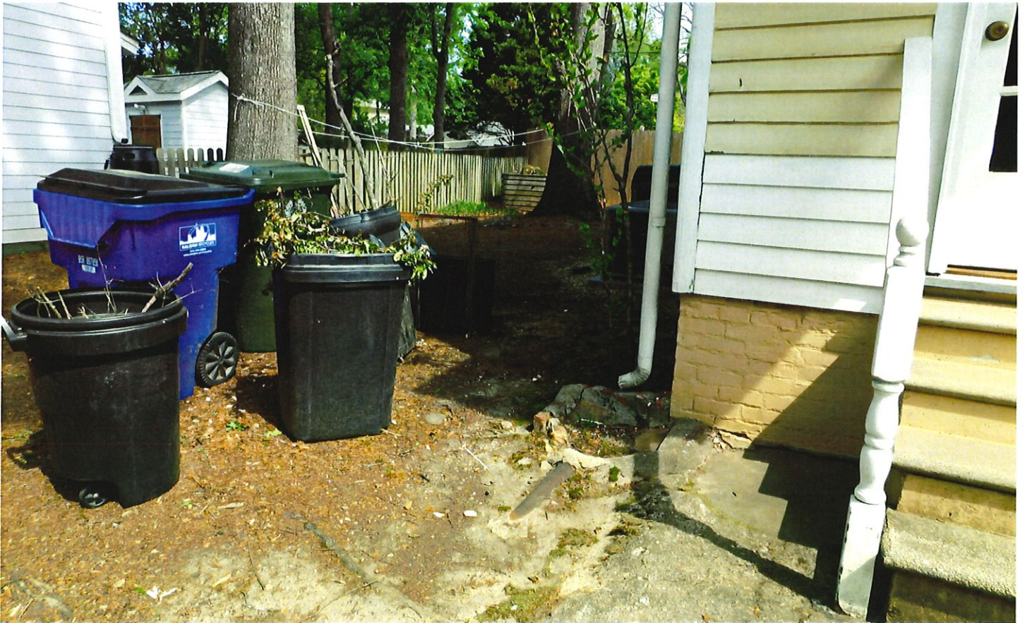
3 SOUTHWEST CORNER OF EXISTING HOUSE
