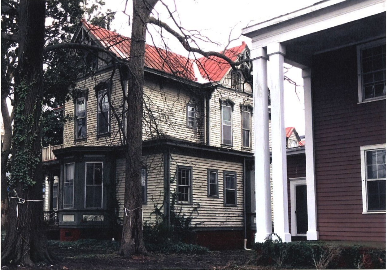
Existing Northeast Facade
