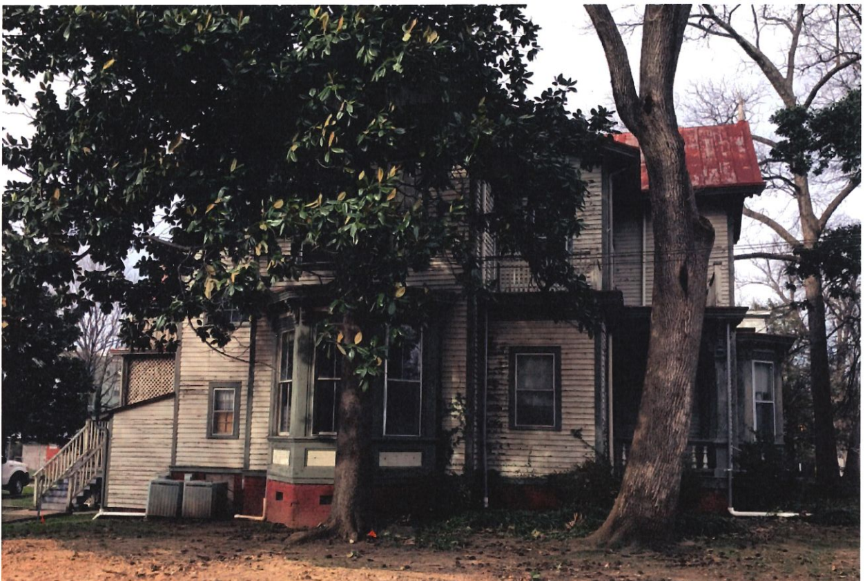
Existing South Facade
