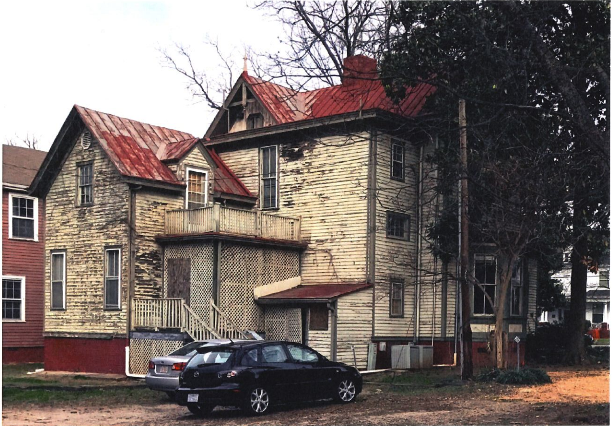
Existing Northwest Facade
