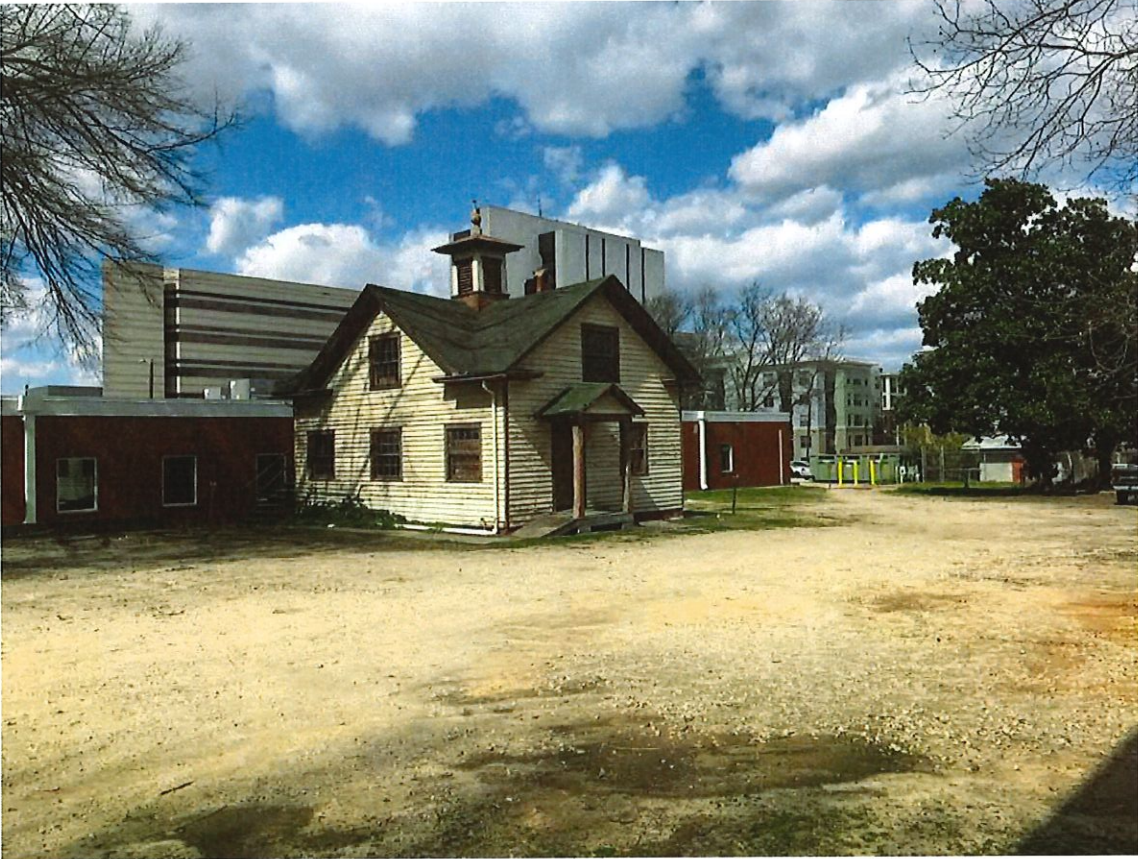
Existing North Facade
