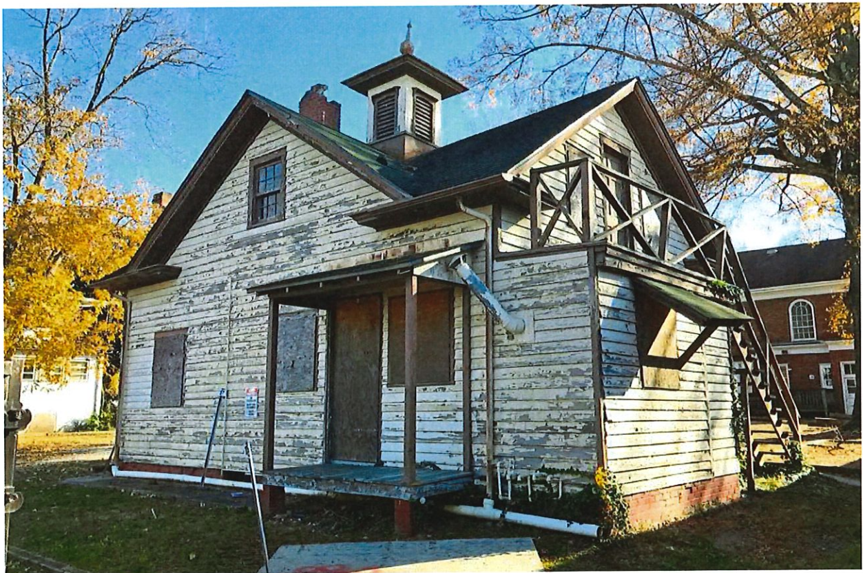
Existing North Facade
