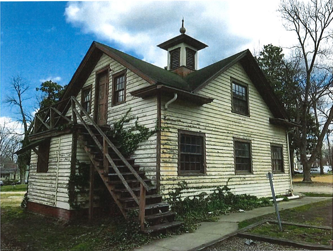
Existing Southwest Facade
