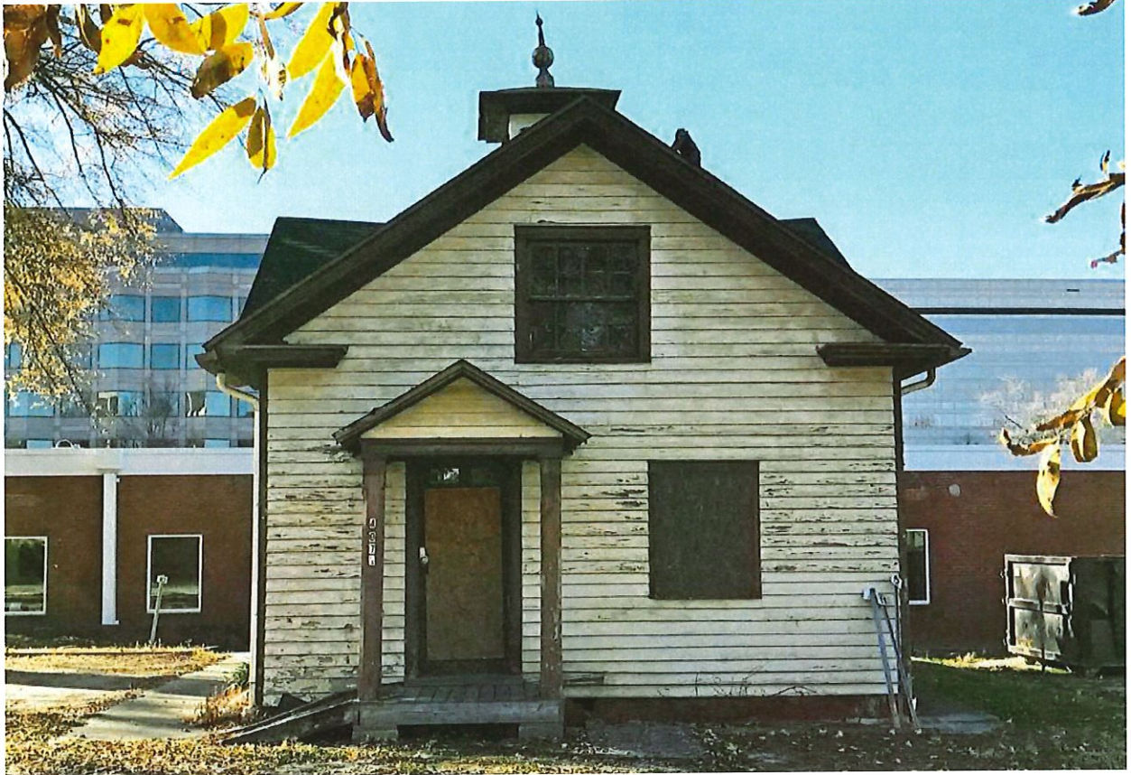
Existing Blount Street Facade - East
