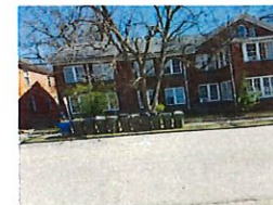
Fascia Repair and Painting
