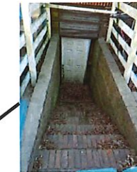
Cellar Door Installation Location
