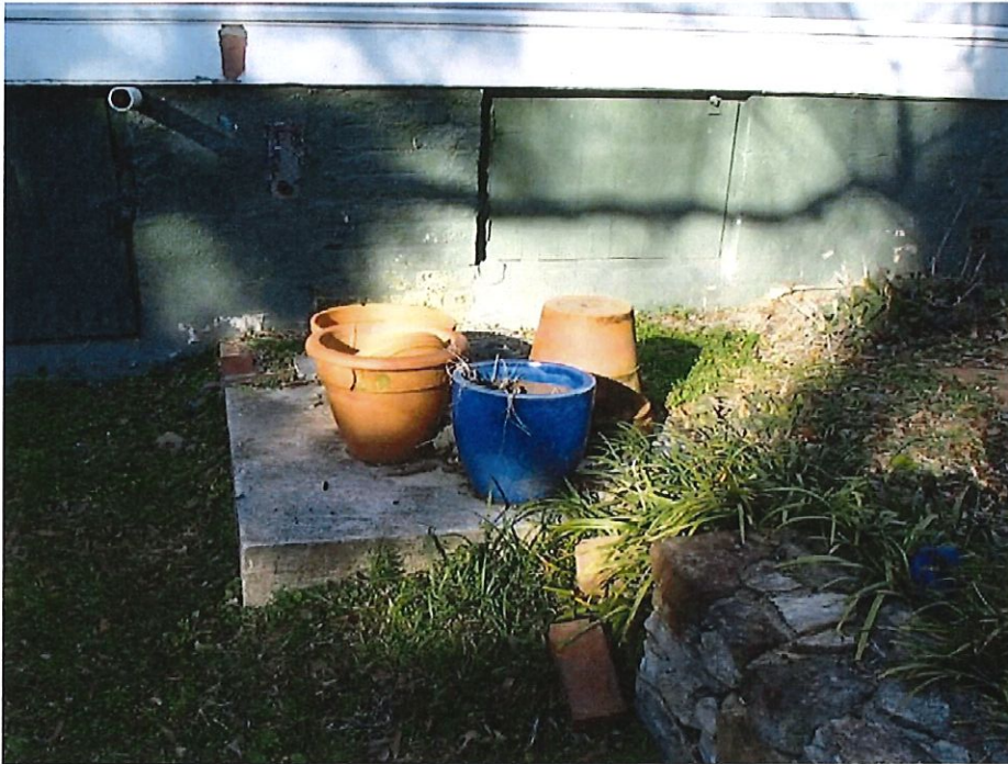
8 Concrete pad to be removed
