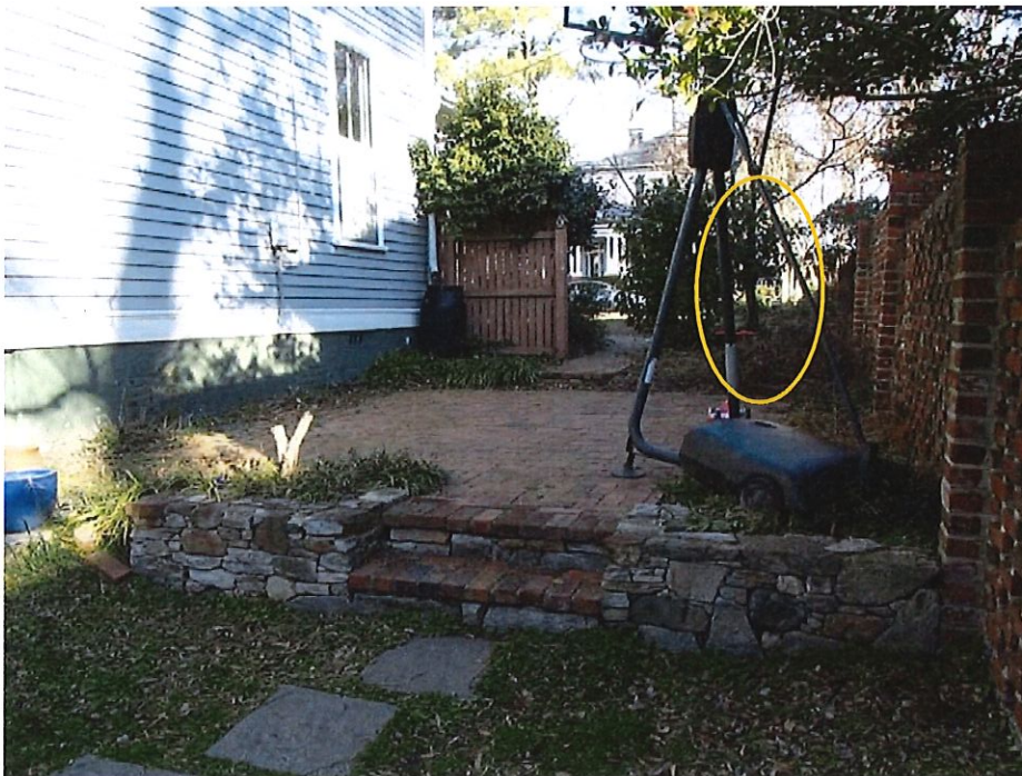
7: existing upper patio; no changes except replacing flowers with grass; gardenia to be removed is highlighted
