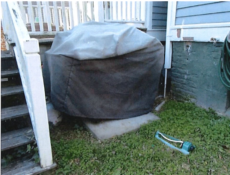
9 Concrete pad (under grill) to be removed
