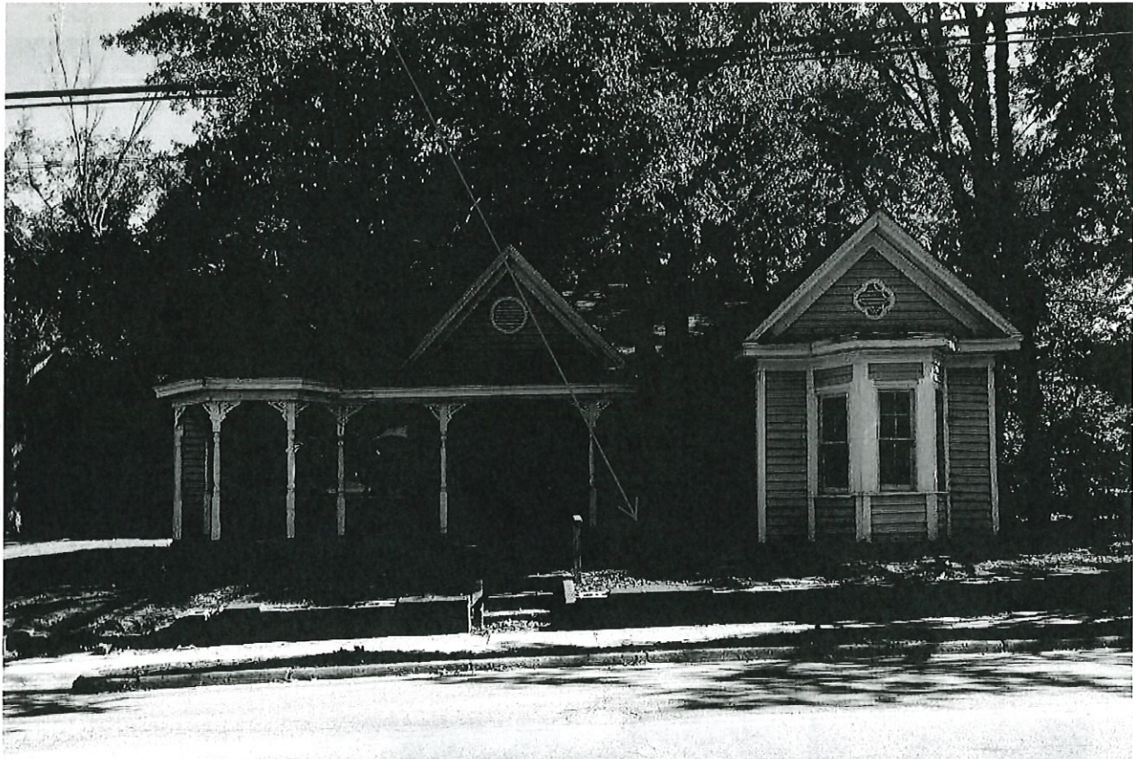
Main (West) Facade
