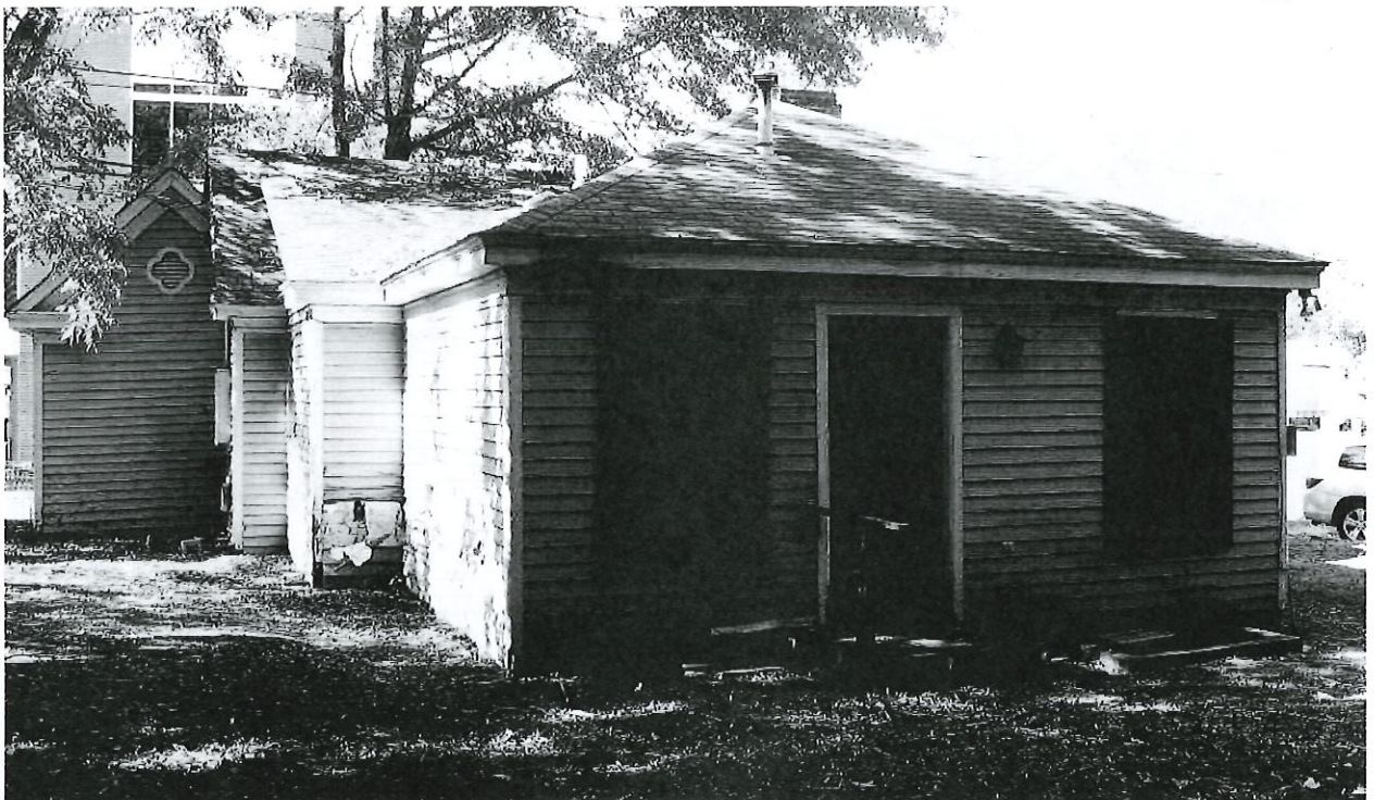
East (Rear) Facade
