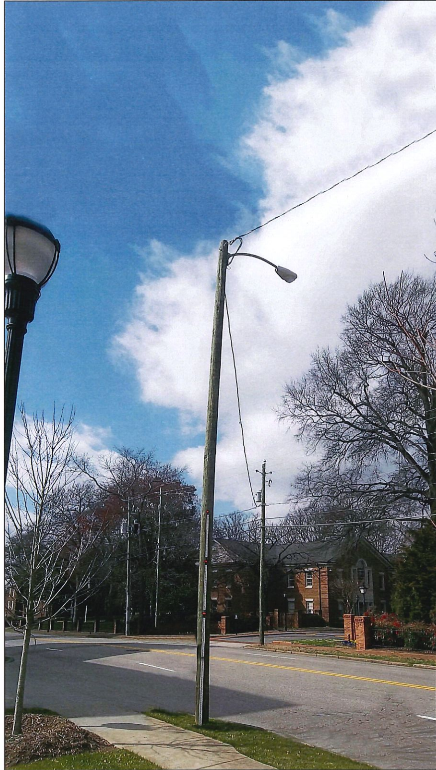
EXISTING PHOTOGRAPHIC VIEW
