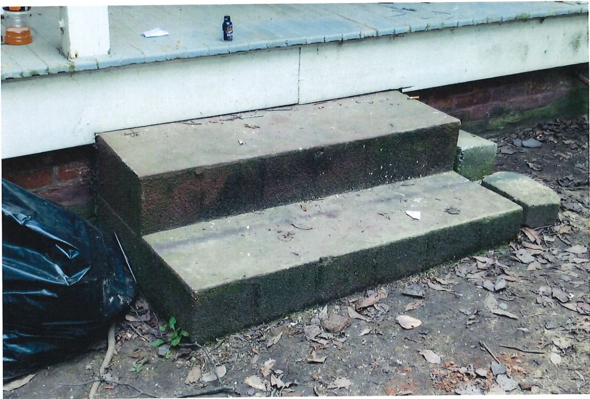
NON-ORIGINAL BACK PORCH STEPS (NORTH SIDE OF HOUSE)
