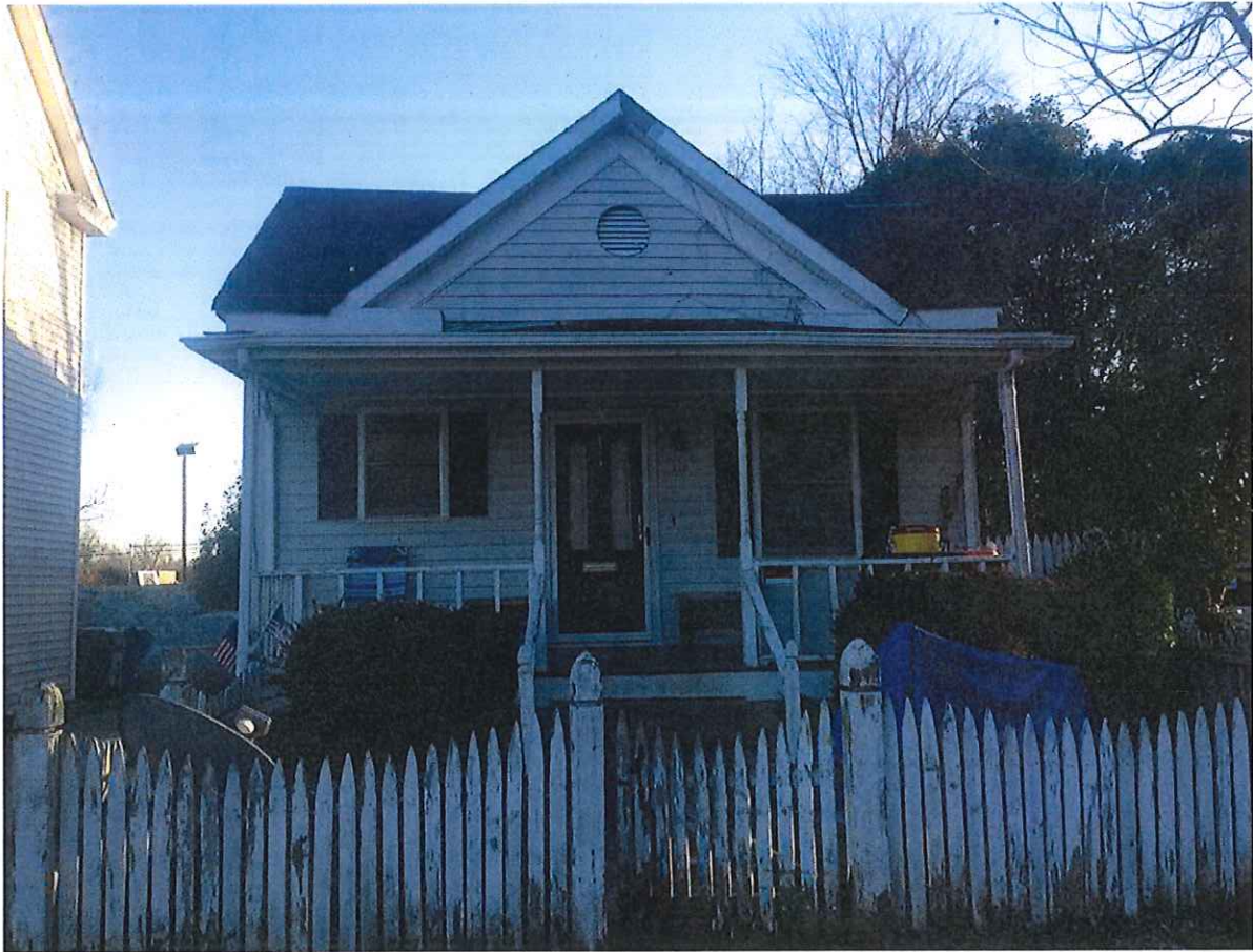
Front of existing house, looking from the north.
