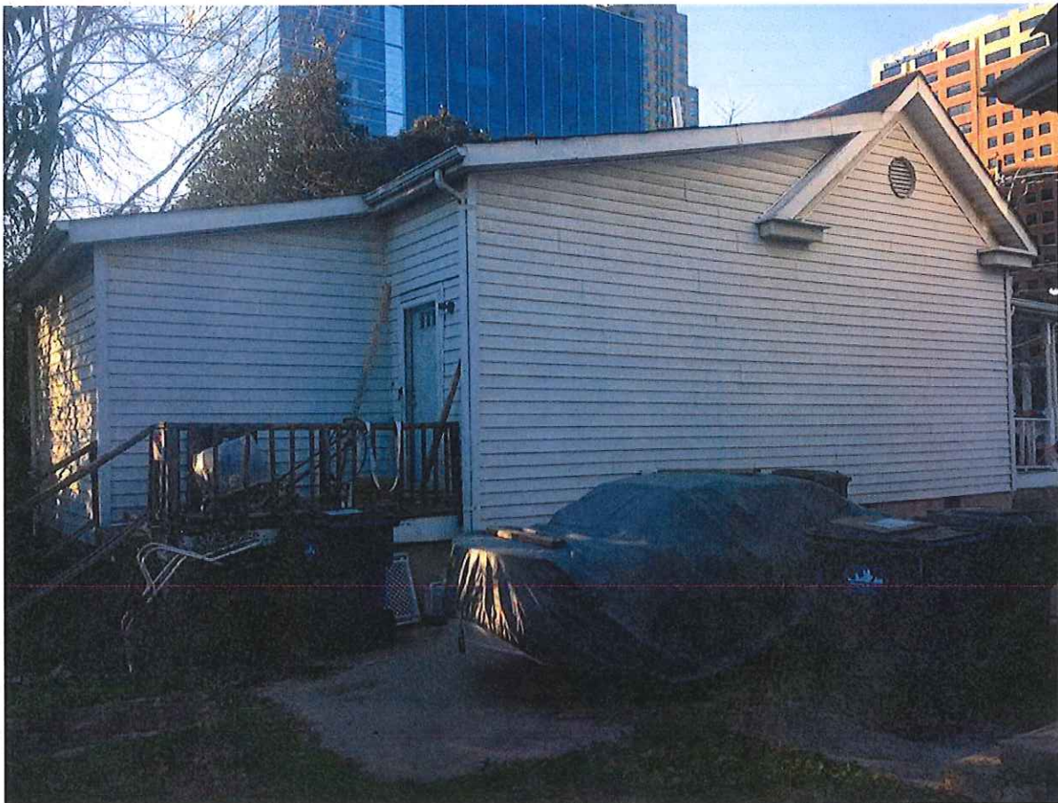
Rear of existing house, looking from the southeast. Bump out addition off back to be removed.
