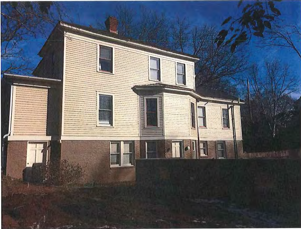
South side of house
