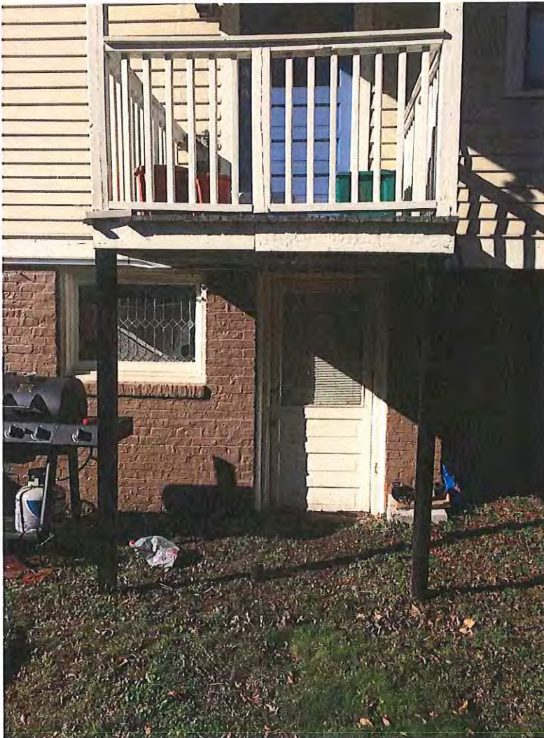
East side of house basement
