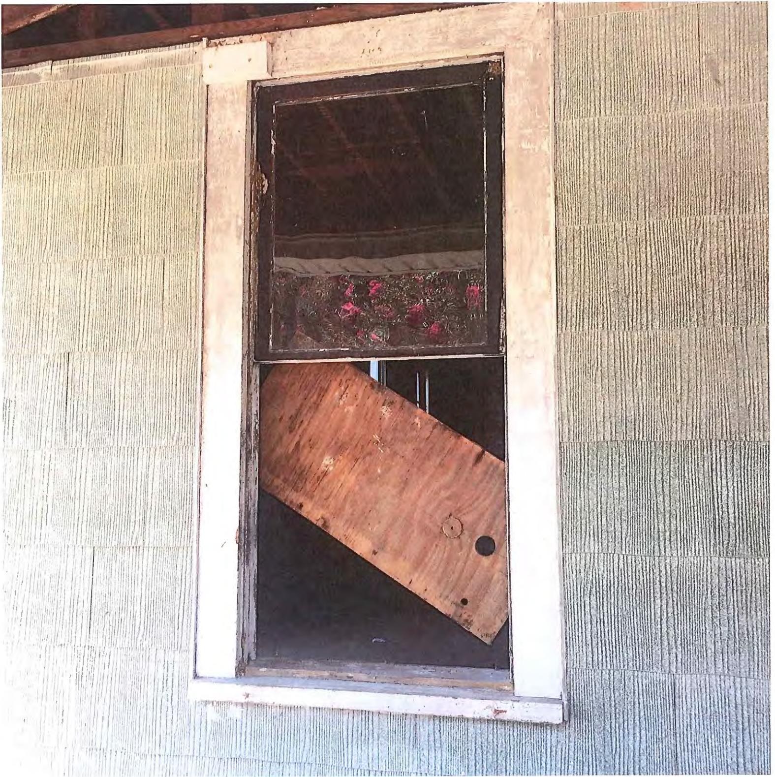
East Window South
