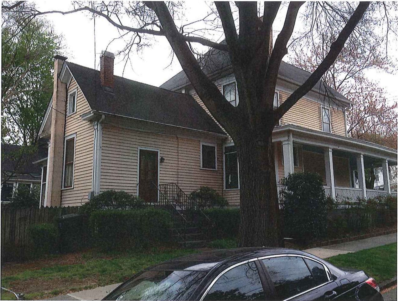
View of the back of the house on East St.
