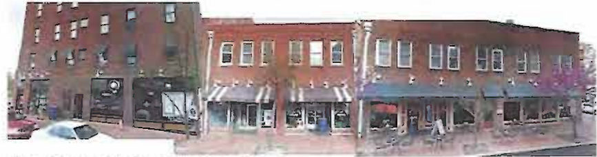
Photos of elevation above for reference and completeness
