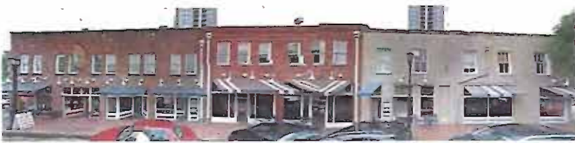
Photos of elevation above for reference
