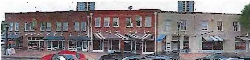
Photos of elevation above for reference
