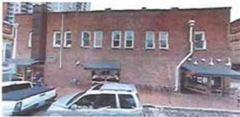
Photos of elevation above for reference
