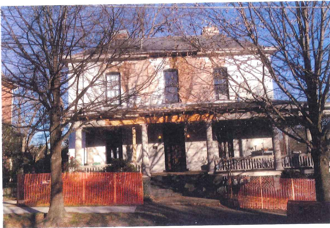
Front of 404 Elm Street facing Elm Street
