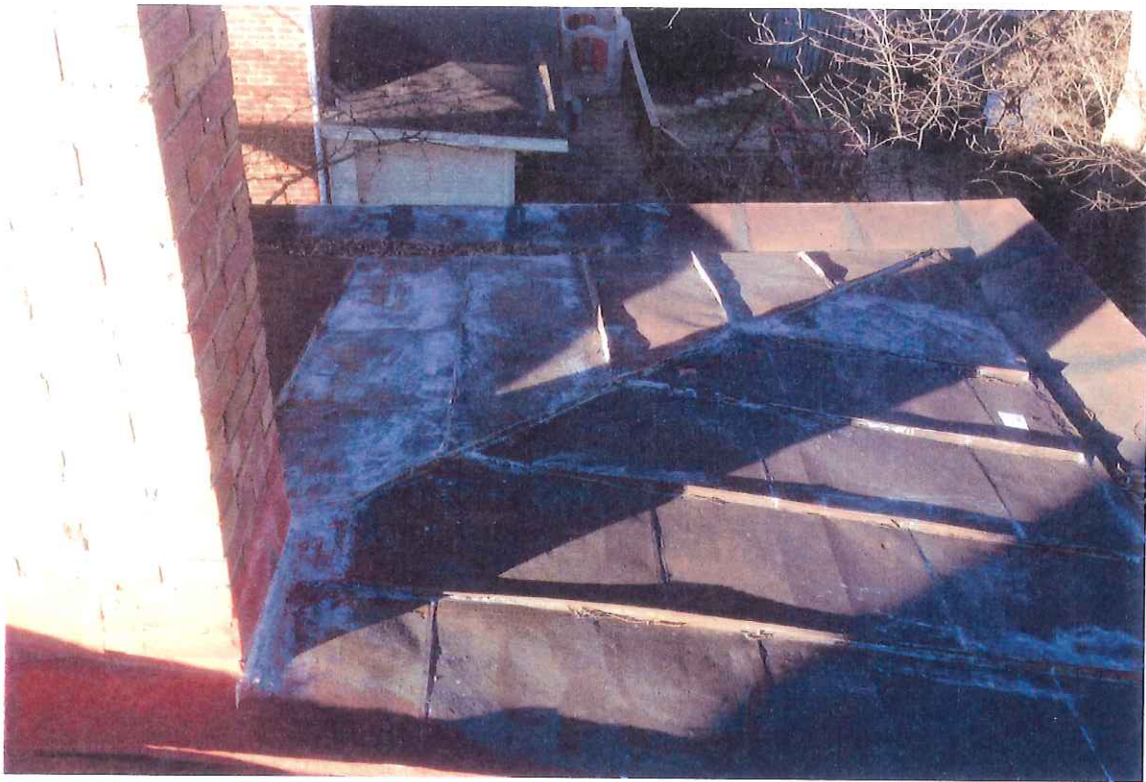
standing-seam metal roof on back 2-story addition added in early 1950's
