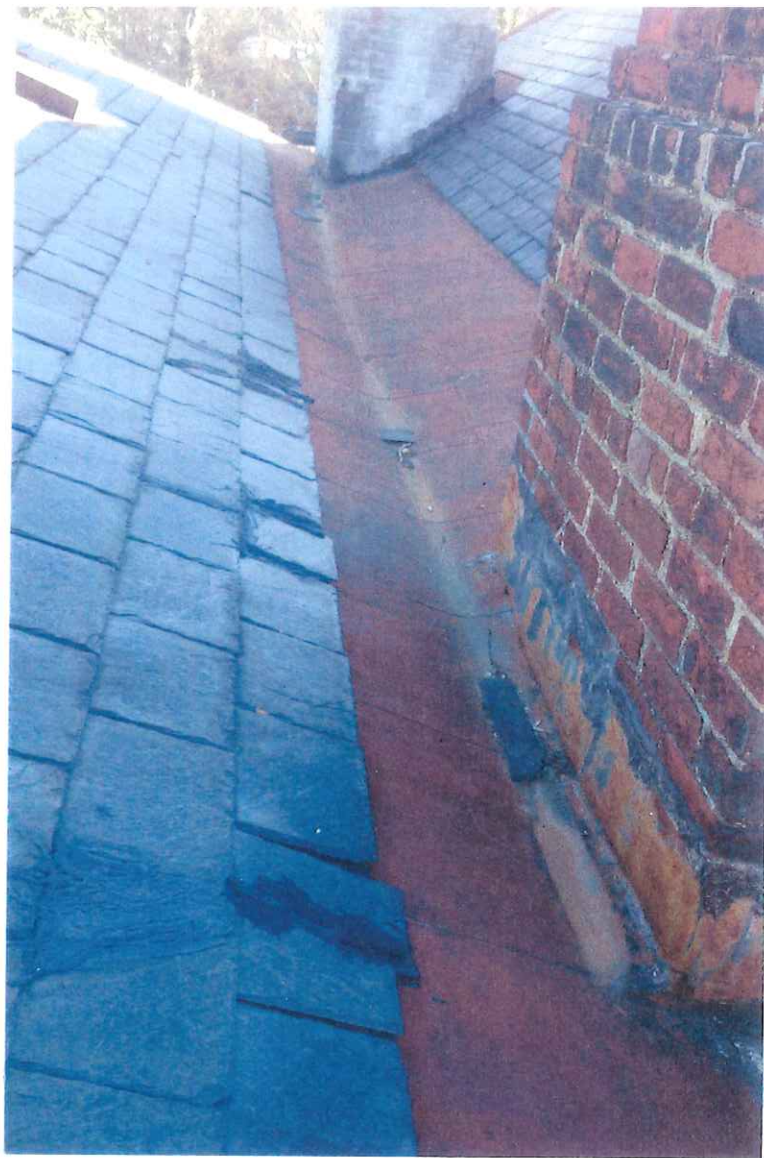
metal cricket between slate roofs, showing chimneys
