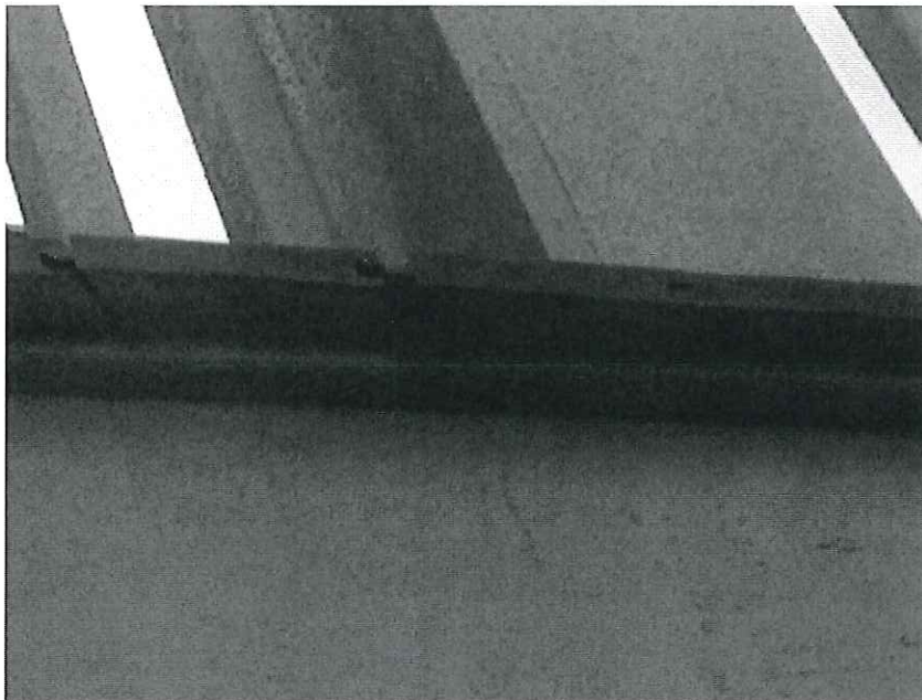
upper deck/porch (photo taken from below)
