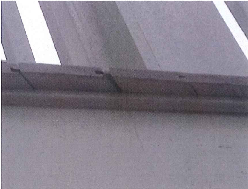
upper deck/porch (photo taken from below)
