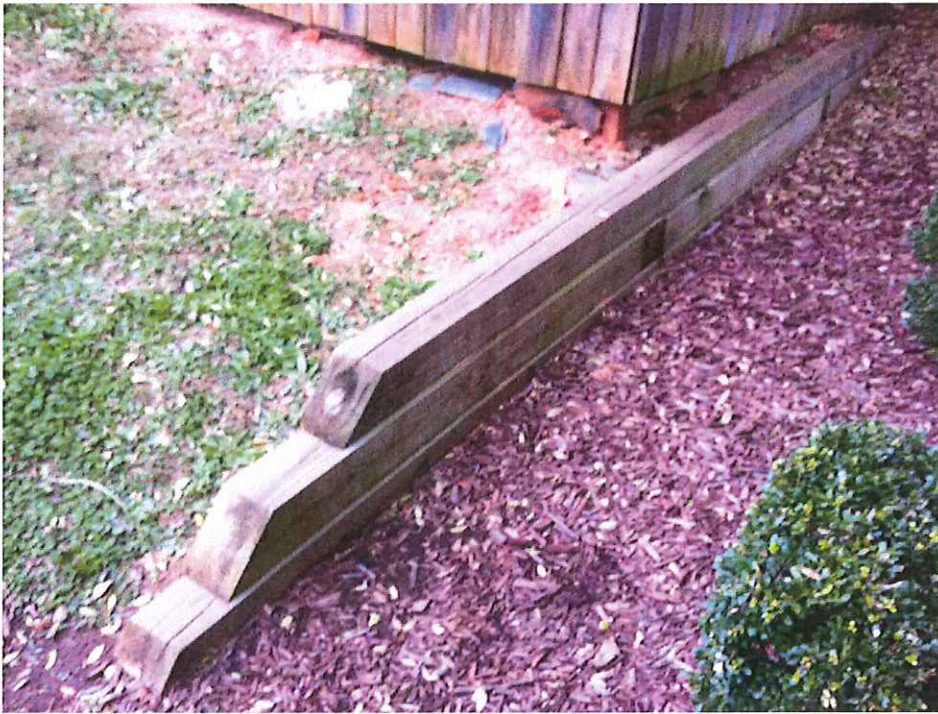
Existing retaining wall that will be
