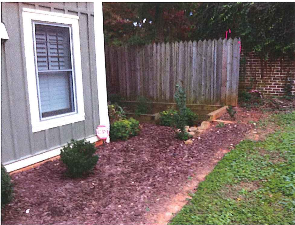
This is the where retaining wall will
