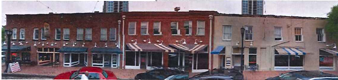
Photos of elevation above for reference
