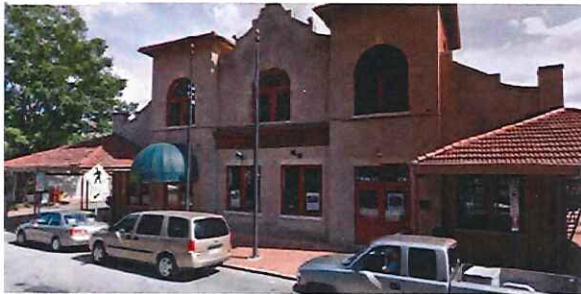
Current photo of elevation above
