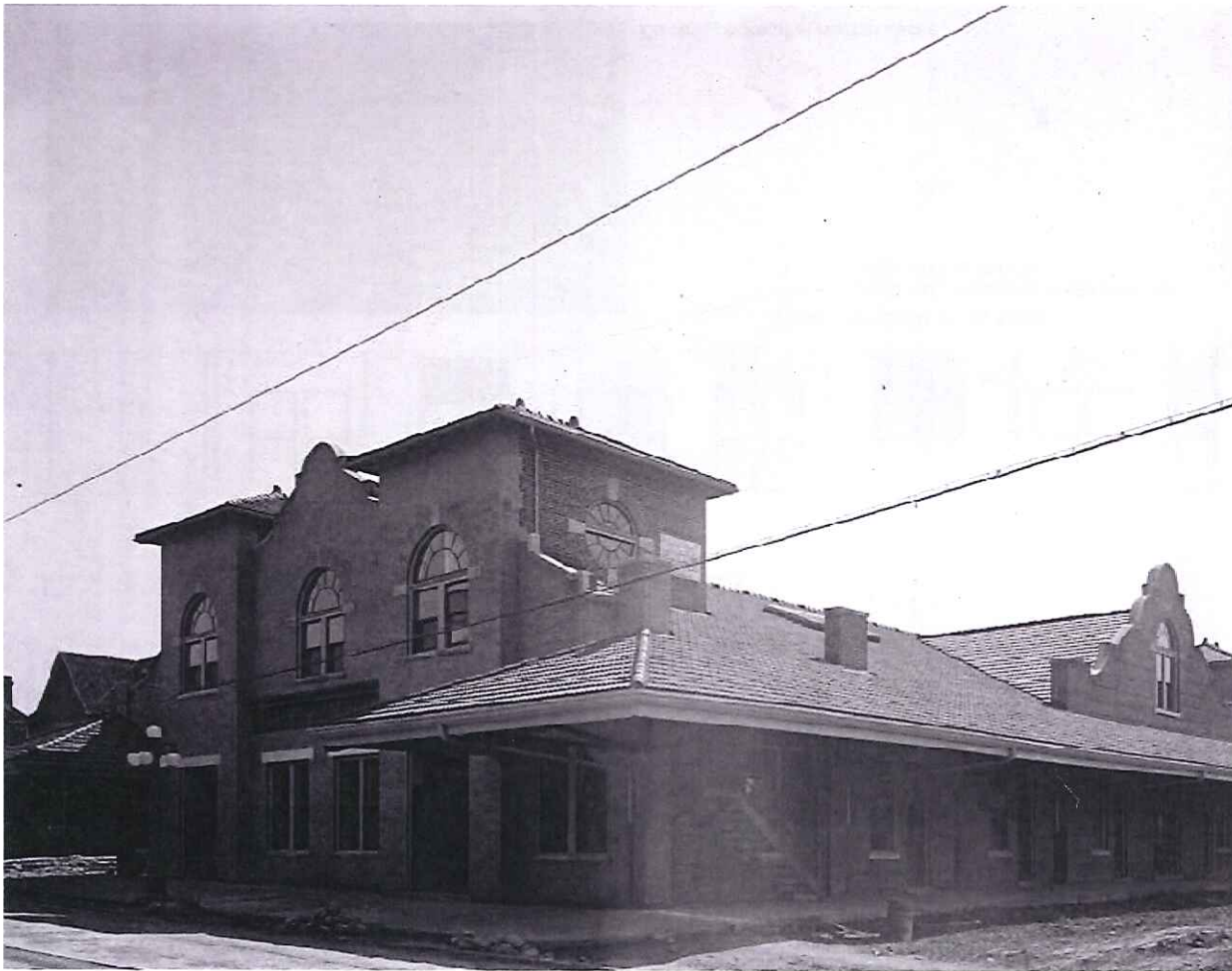
Historic photos showing detailed contrast between trim and windows/doors
