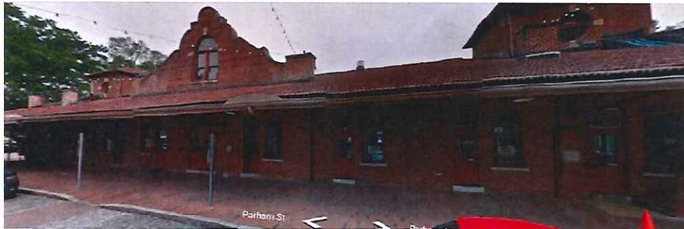
Current photo of elevation above
