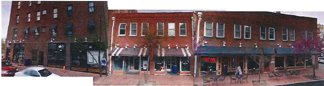
Photos of elevation above for reference and completeness
