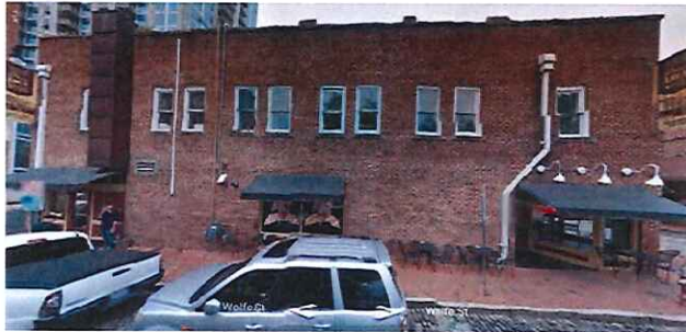
Photos of elevation above for reference
