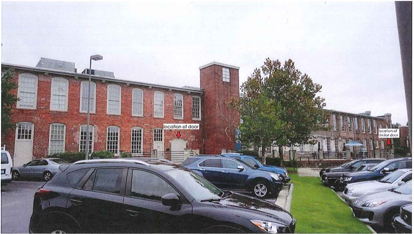
1111 Haynes West Facade
