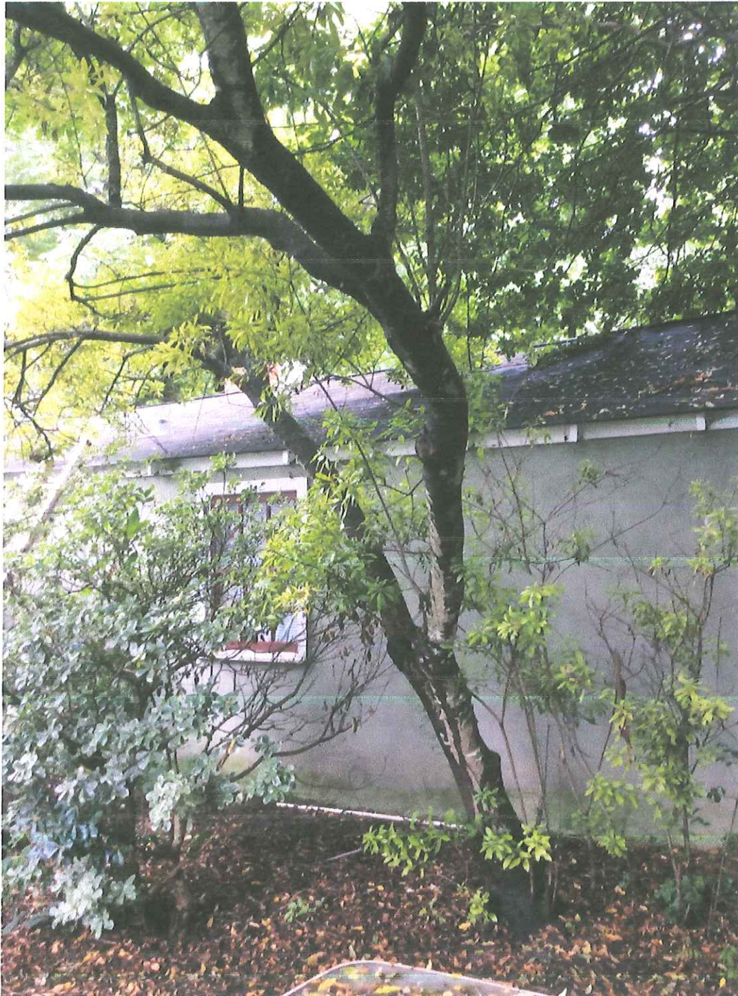
Wax myrtle to be removed, struggling and too close to the structure.
