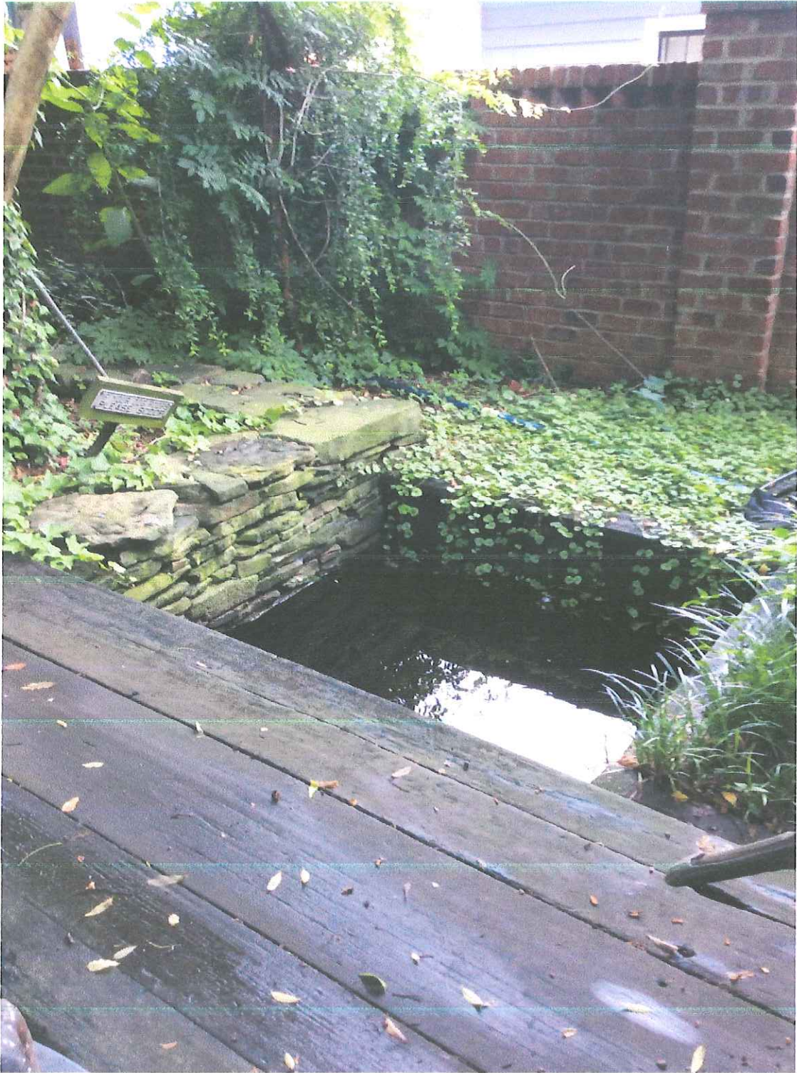
Pond to be filled in, bridge to be removed, and stone wall to remain
