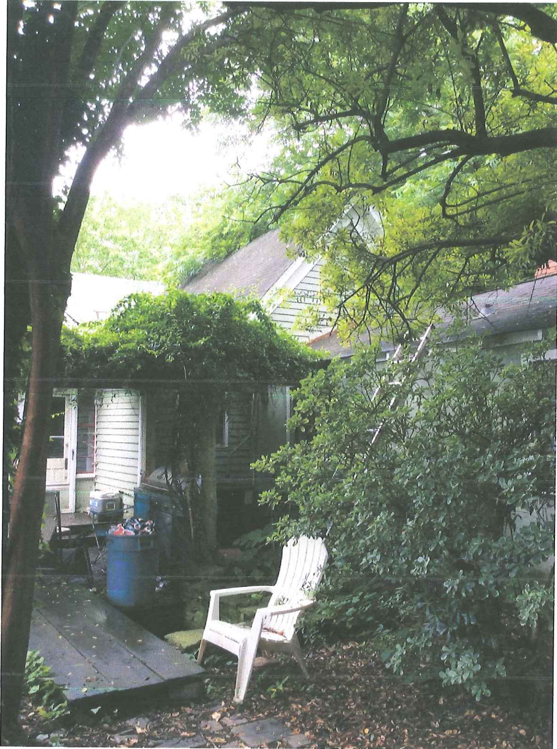
Portion of trellis that attaches to the existing rear addition to be removed
