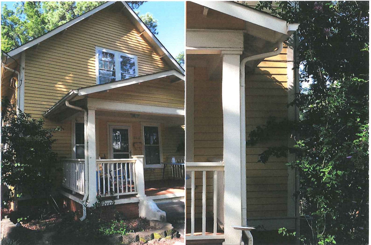
Photo #1 – 913 South Street – K-style gutters installed onto fascia with exposed rafter tails
