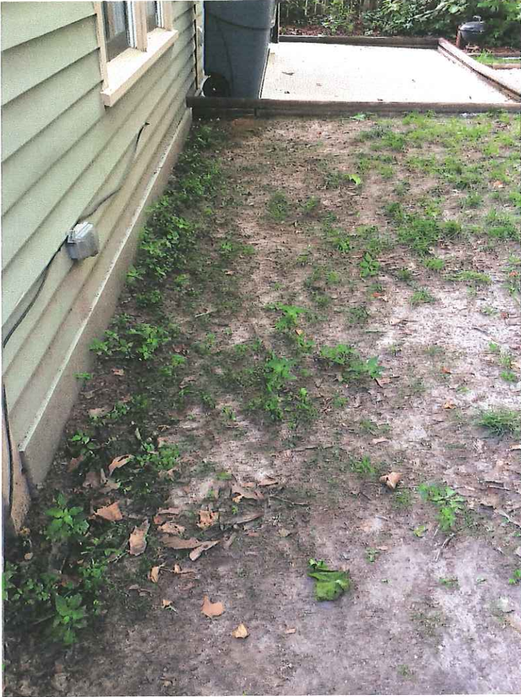
Photo #7 – Existing rear of house
