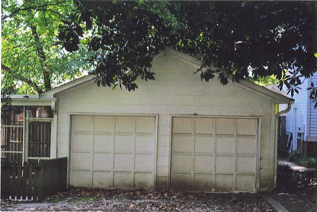
Up-close of existing garage front elevation and current overhang + eave condition
