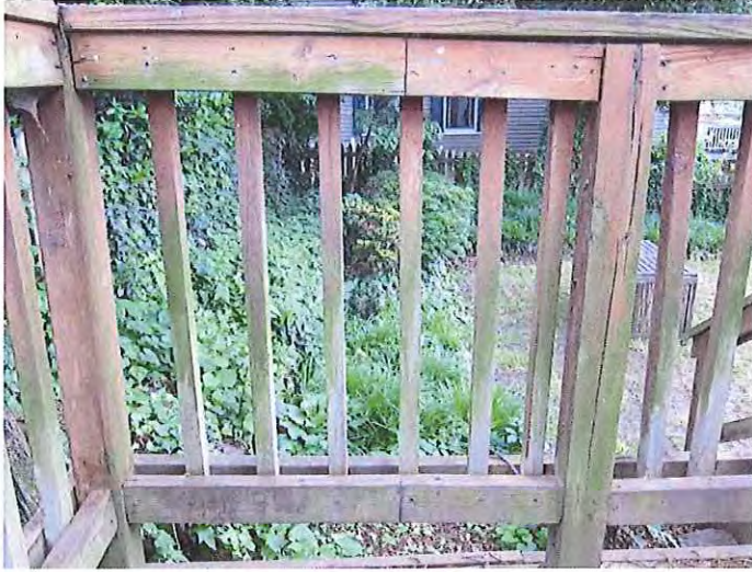
Figure 12: Image of railing to be replaced
