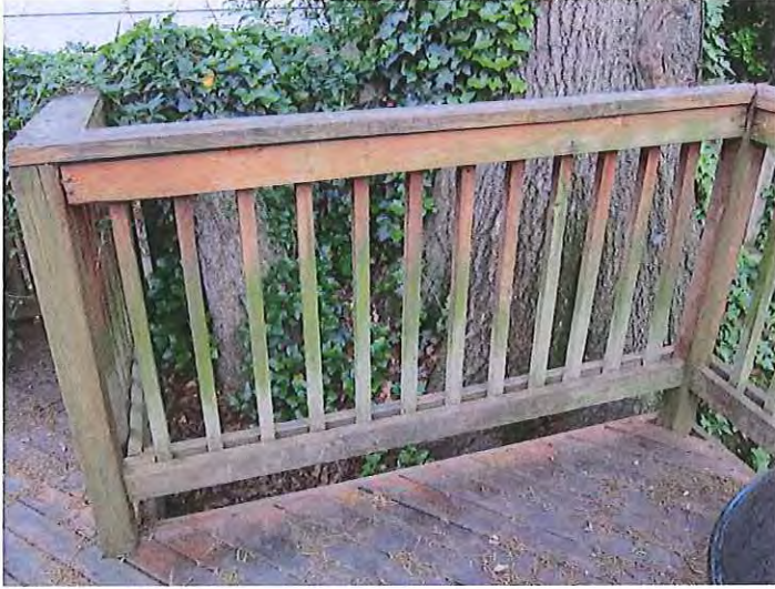
Figure 15: Image of railing to be replaced
