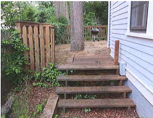
Figure 7: Deck and stairs: taken looking towards back of property
