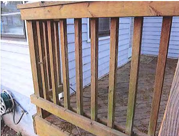
Figure 14: Image of railing to be replaced
