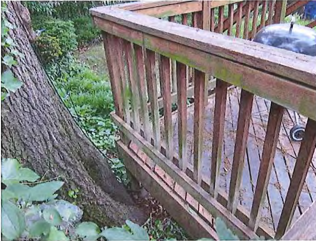
Figure 16: Image of railing to be replaced
