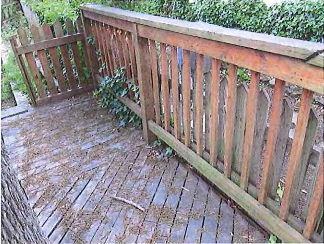
Figure 9: Additional angle of deck closest to neighbor
