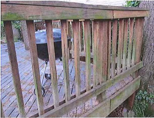
Figure 13: Image of railing to be replaced
