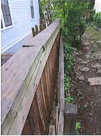
Figure 18: Image of railing to be replaced
