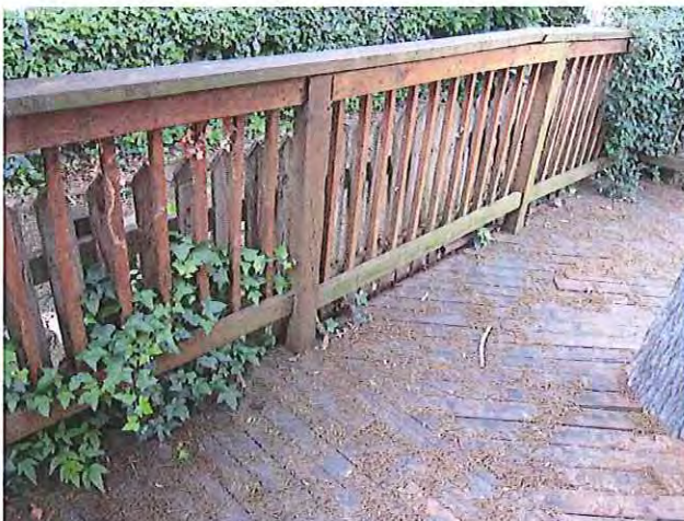
Figure 8: Deck edge closest to neighbor
