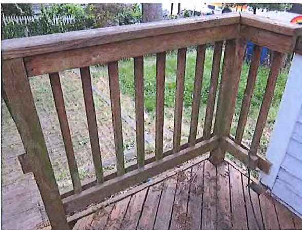
Figure 17: Image of railing to be replaced
