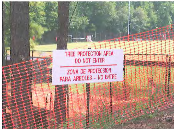
Figure 1. Tree protection zone. A protected zone preserves roots and soil and keeps branches clear of contact with construction equipment and materials.
